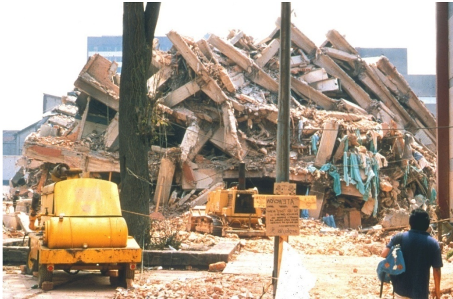
Figure 4-5 Collapse due to connection failures in the 1985 Michoacán (Mexico) Earthquake (Courtesy of Mete Sozen).
