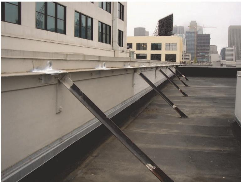
Figure 6-4      Example of parapet bracing (FEMA, 2012).
