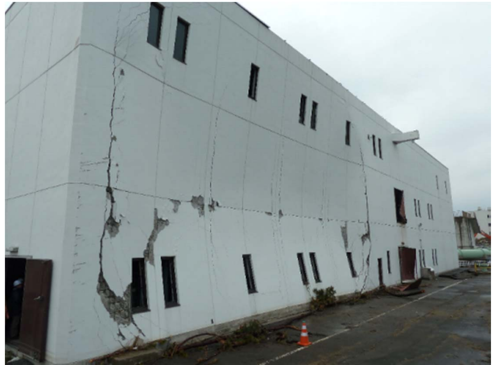
A filtration plant
