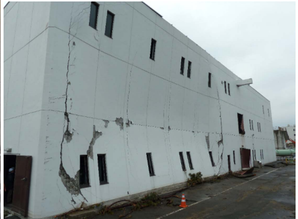
A filtration plant
