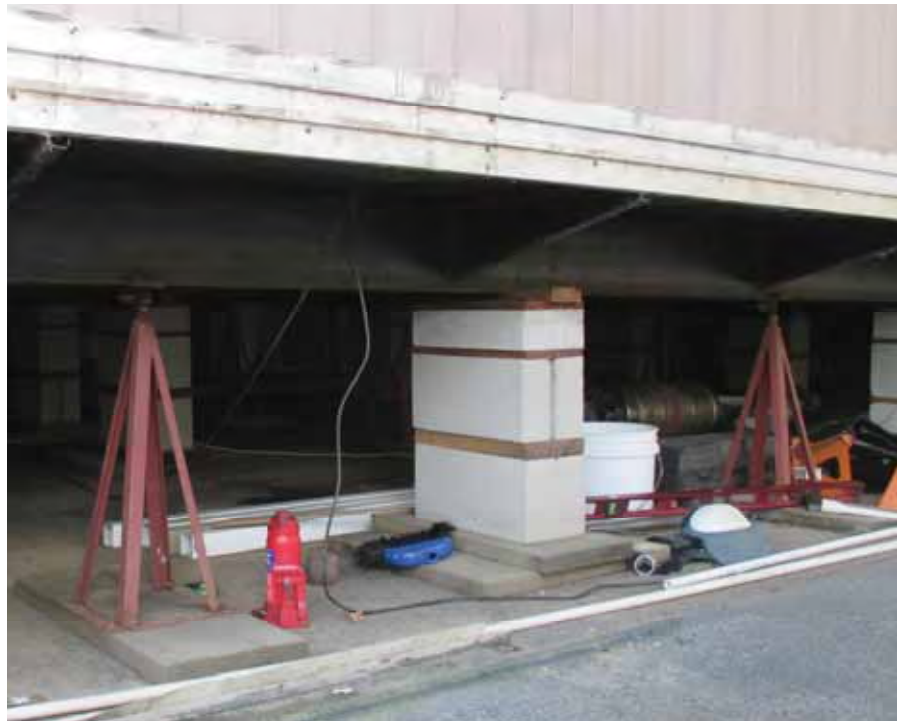
Figure 8-4 Steel gravity piers interspersed with masonry piers during home reinstallation.
