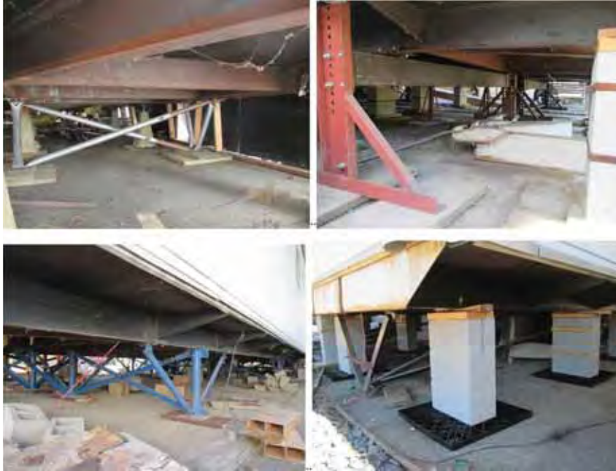
Figure 8-11 “Diagonally braced” ERBS on homes requiring reinstallation.
