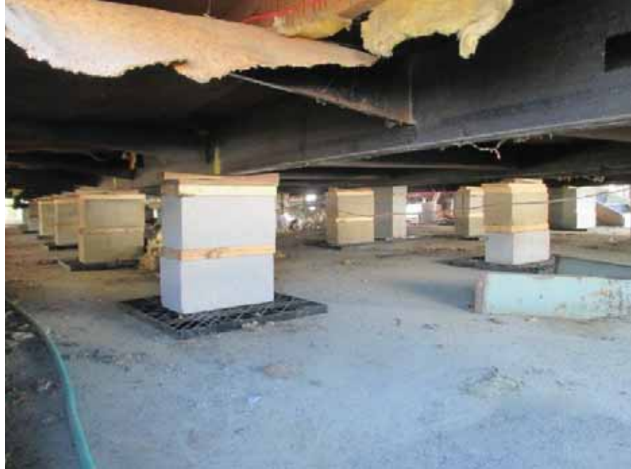
Figure 8-3 Typical dry-stacked masonry gravity piers, with interspersed wood blocks.
