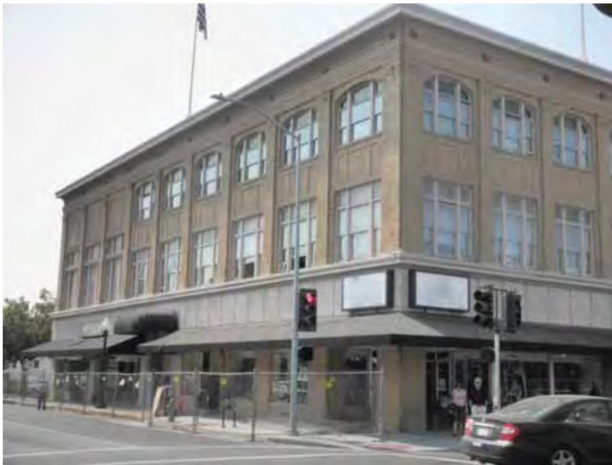
Figure 4-19 Exterior view of building.
