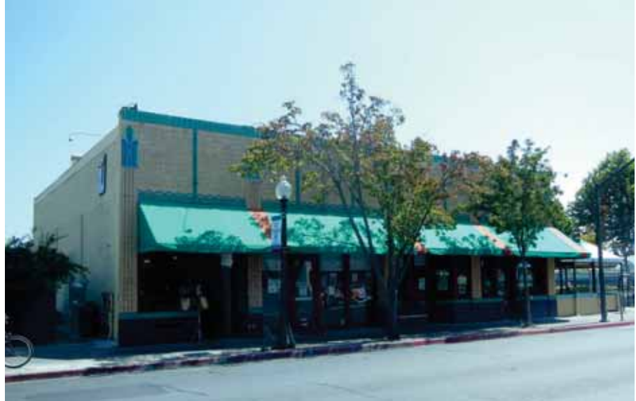
Figure 4-89 Building elevation from Main Street.
