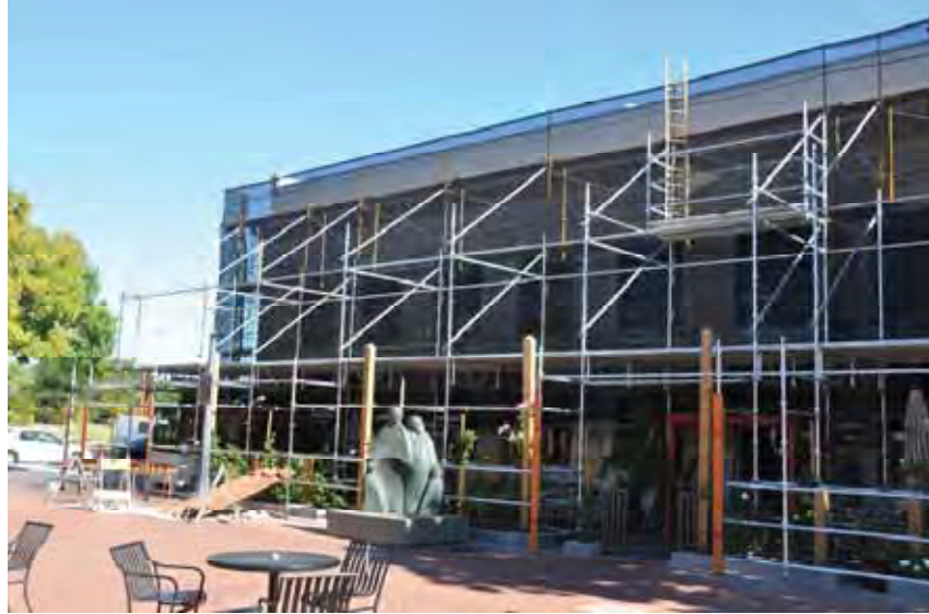
Figure 12-6 Replacement scaffolding following the windstorm (photo by Fred Turner).
