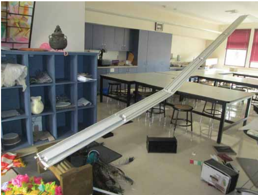
Figure 6-5 Damaged light fixtures in Napa Valley Language Academy (photo by Quattrocchi Kwok Architects).
