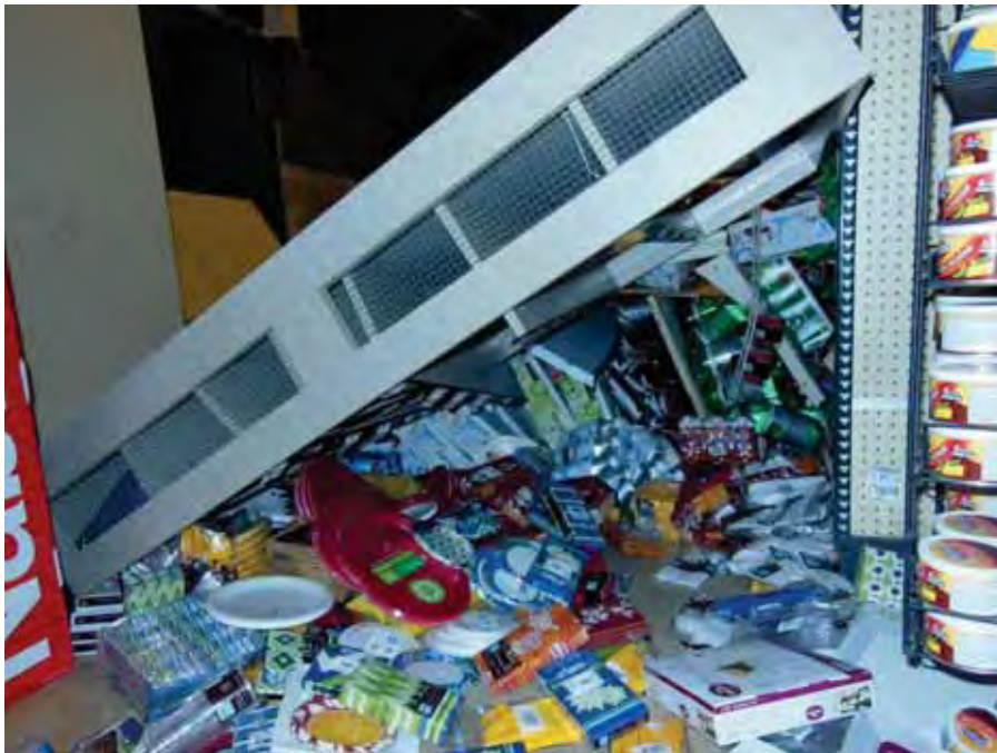
Figure 4-31 Overturned store fixture, loss of contents.
