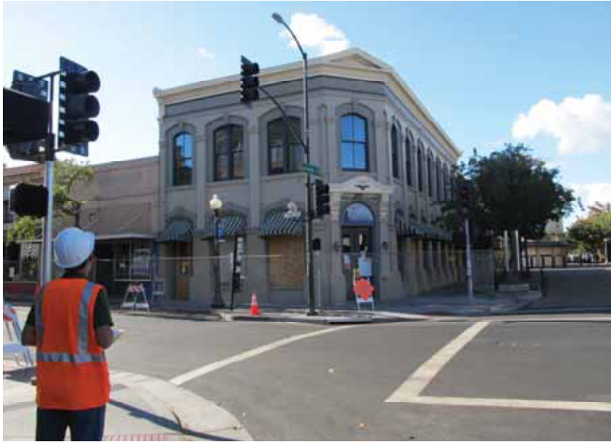
Figure 12-1 A building with an UNSAFE placard where the fence setback was much less than a 1.5H:1V setback distance.
