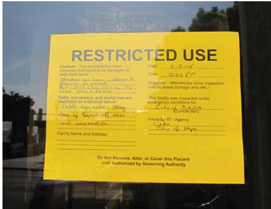
Figure 11-2 A RESTRICTED USE tag with restrictions noted as “Public may enter. Stay clear of taped off areas and construction.”
