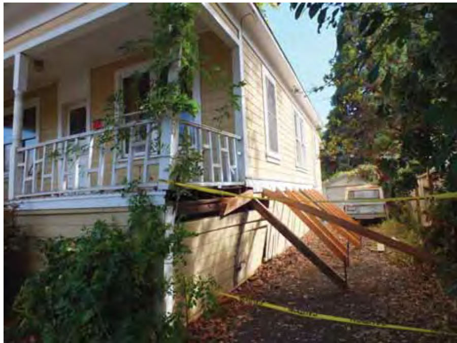
Figure 7-15 Temporary lateral bracing at cripple wall.
