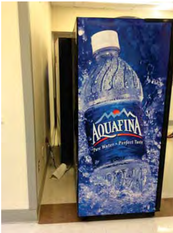
Figure 5-20 Unanchored vending machine in BLD-01656 shifted over 12 inches.
