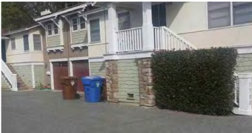
Figure 7-20 Elevated duplex homes.
