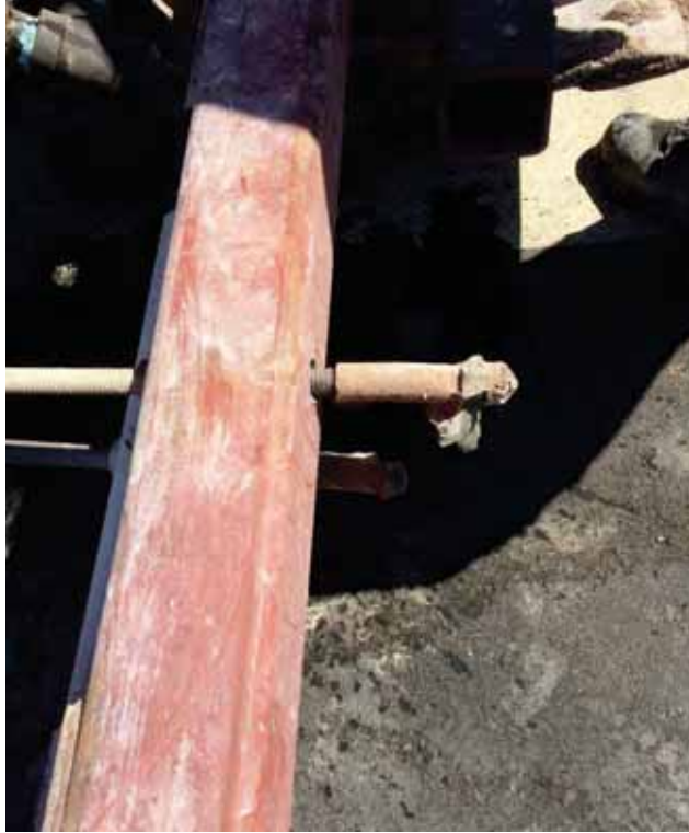
Figure 4-58 Close-up of steel tube and masonry anchor at corner cupola.
