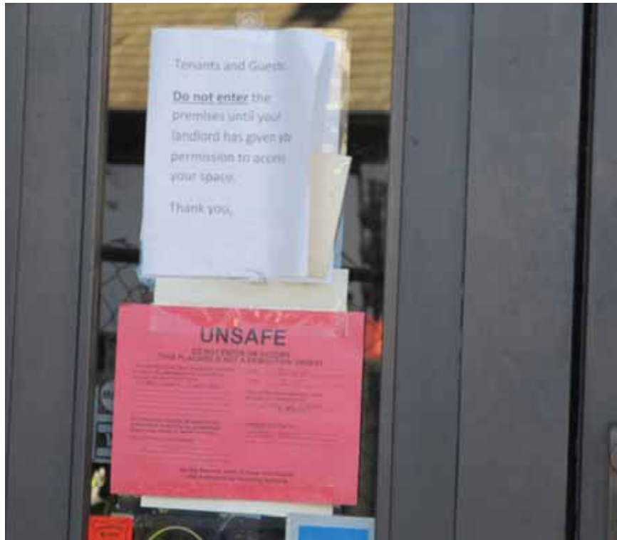
Figure 11-6 An UNSAFE placard with an adjacent inconsistent placard by the owner.
