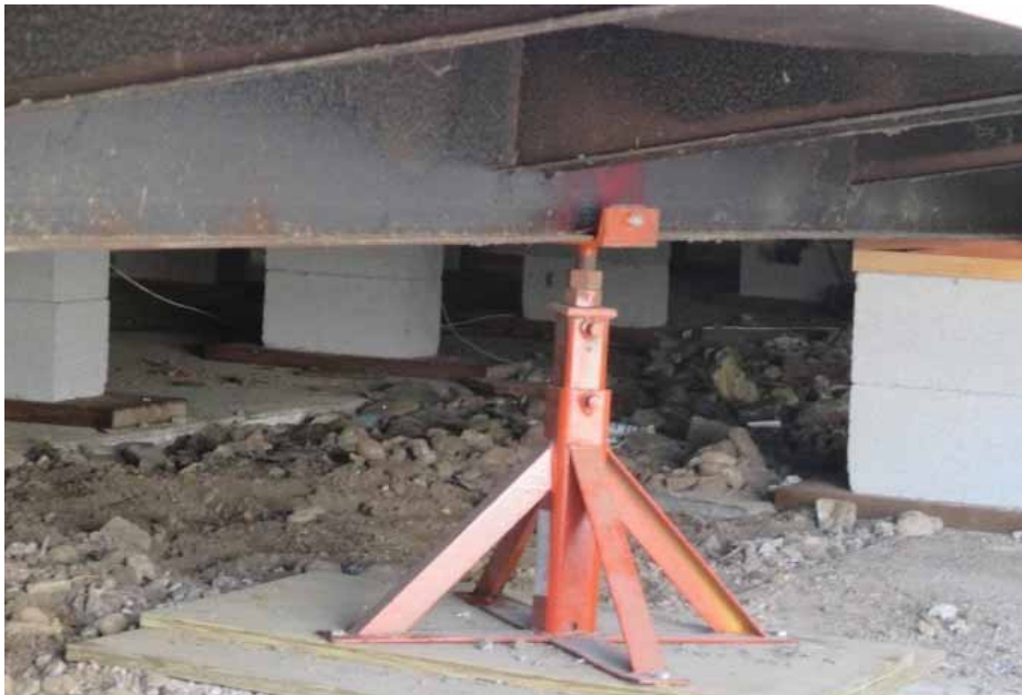
Figure 8-9 New “cantilevered” pier, anchored to supporting plywood panels.
