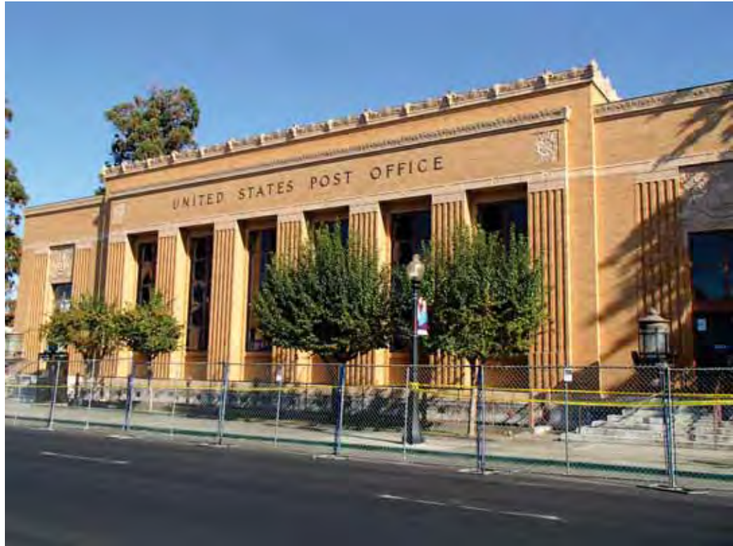
Figure 4-23 Exterior view of building.
