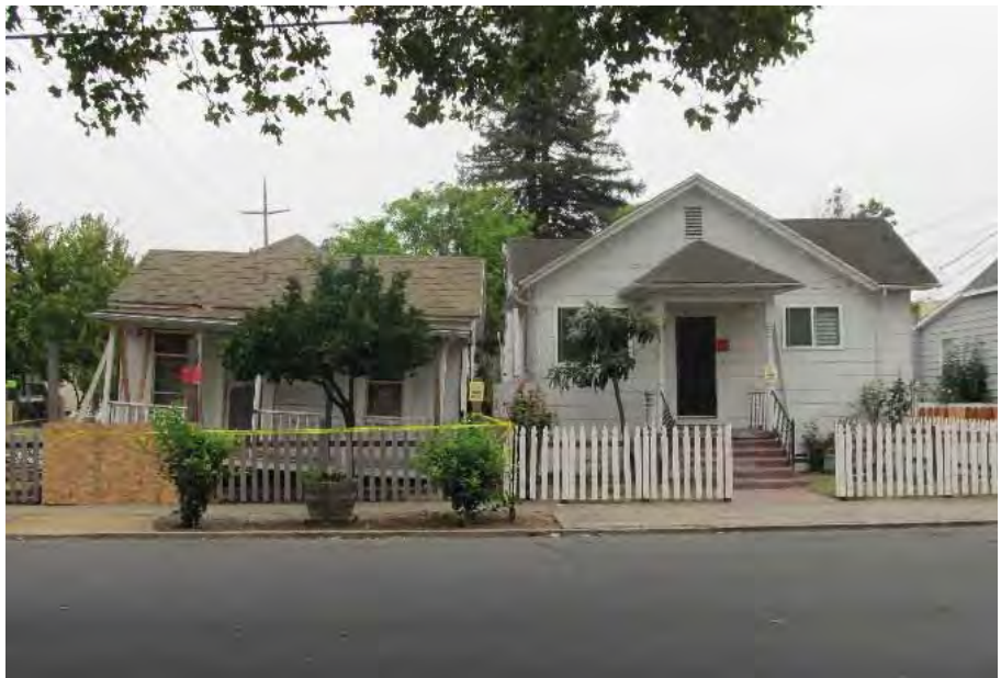
Figure 7-19 Undamaged residence on the right was posted UNSAFE due to risk posed by damaged residence on the left.
