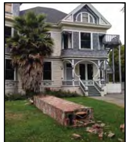
Figure 2: Chimney damaged in the South Napa Earthquake. Photo Credit: Janiele Maffei, CEA
