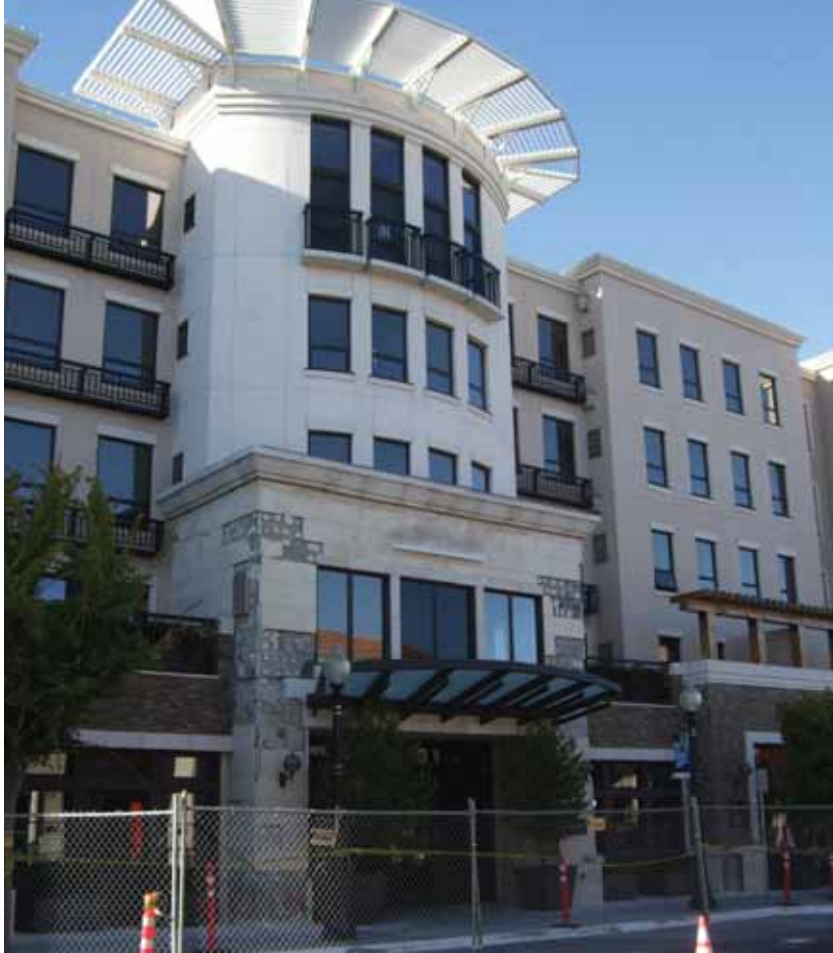
Figure 4-13 Exterior view of building.
