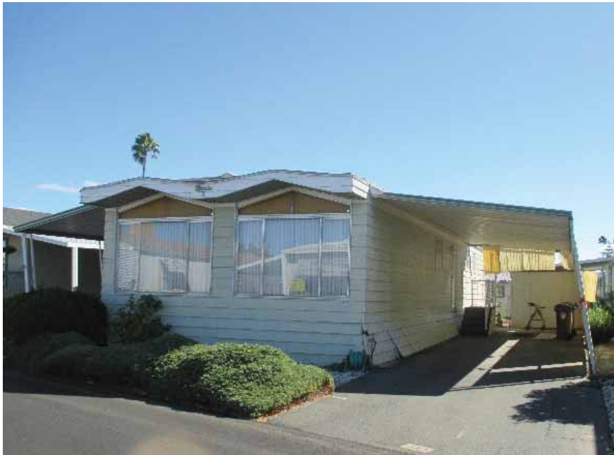
Figure 8-25 Napa Valley MHP home displaced significantly to the east.
