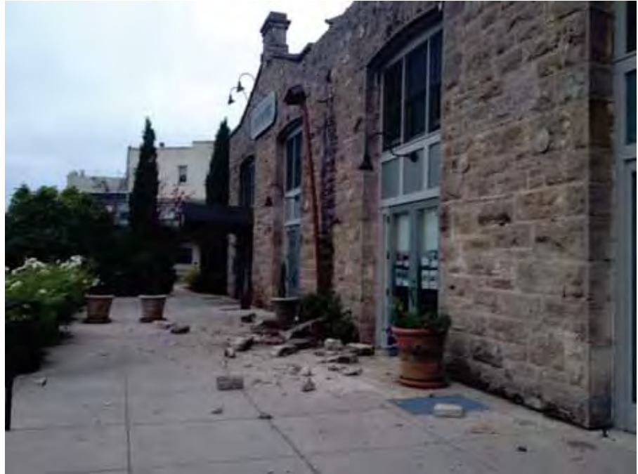
Figure 4-72 Exterior wall on day of earthquake.
