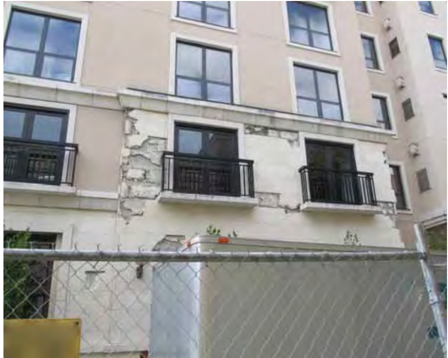
Figure 4-17 Stone masonry veneer, showing where loose units have been removed.
