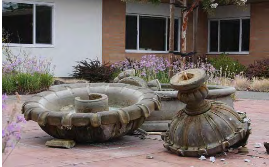
Figure 6-40 Toppled landscape statuary (photo by Quattrocchi Kwok Architects).
