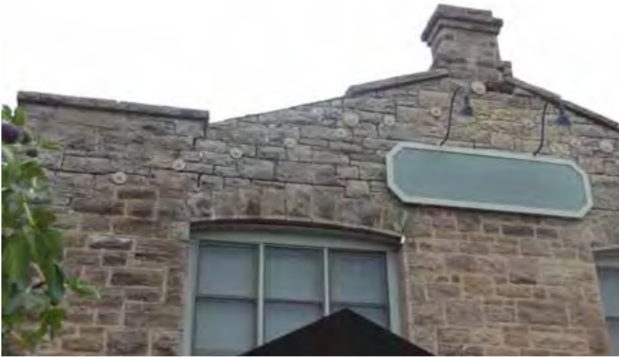
Figure 4-74 Exterior face of parapet wall.
