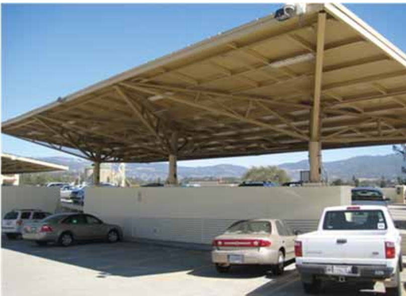
Figure 10-40 Roof-mounted solar canopy on top of parking garage structure. No damage was reported.
