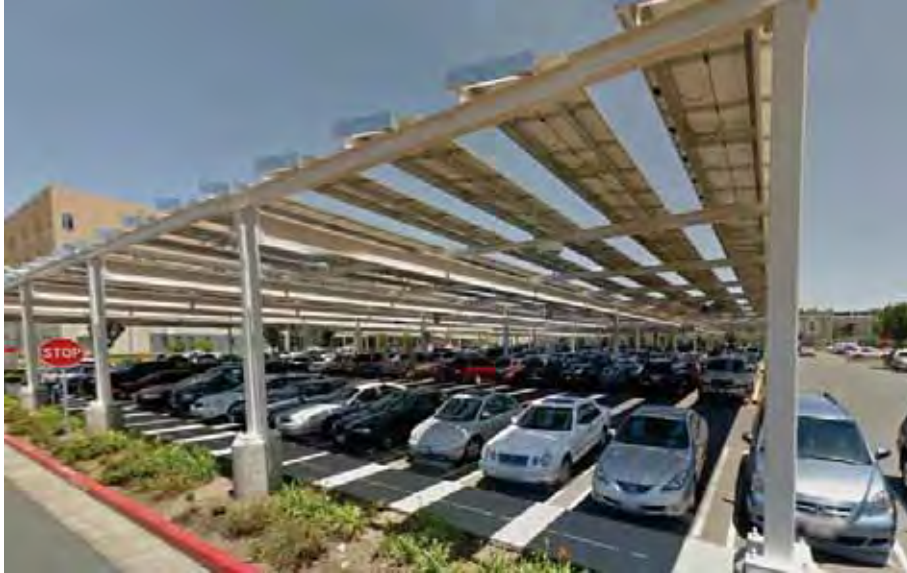
Figure 10-33 Ground-mounted solar canopy over parking lot (photo from Google Street View). No damage reported.
