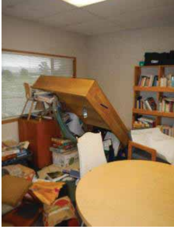
Figure 6-12 Overturned bookcase in Stone Bridge School (photo by Quattrocchi Kwok Architects).
