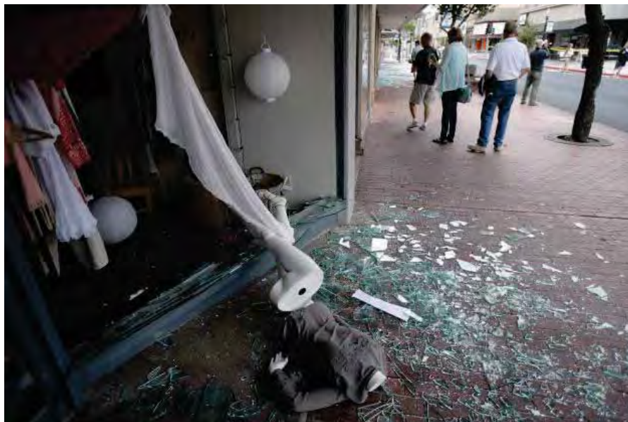
Figure 10-1 Broken glass at open storefront on an unreinforced masonry building.
