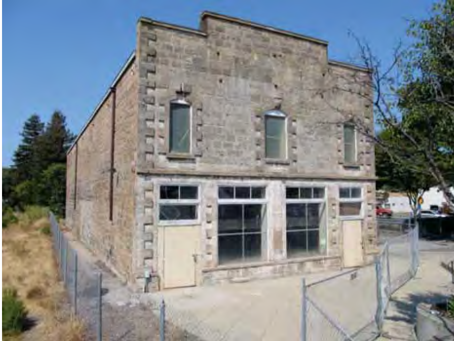
Figure 4-77 View from the southwest showing front façade and fencing.
