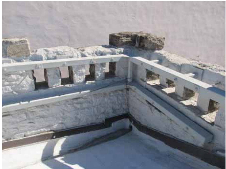
Figure 4-62 Steel tube bracing at parapet.
