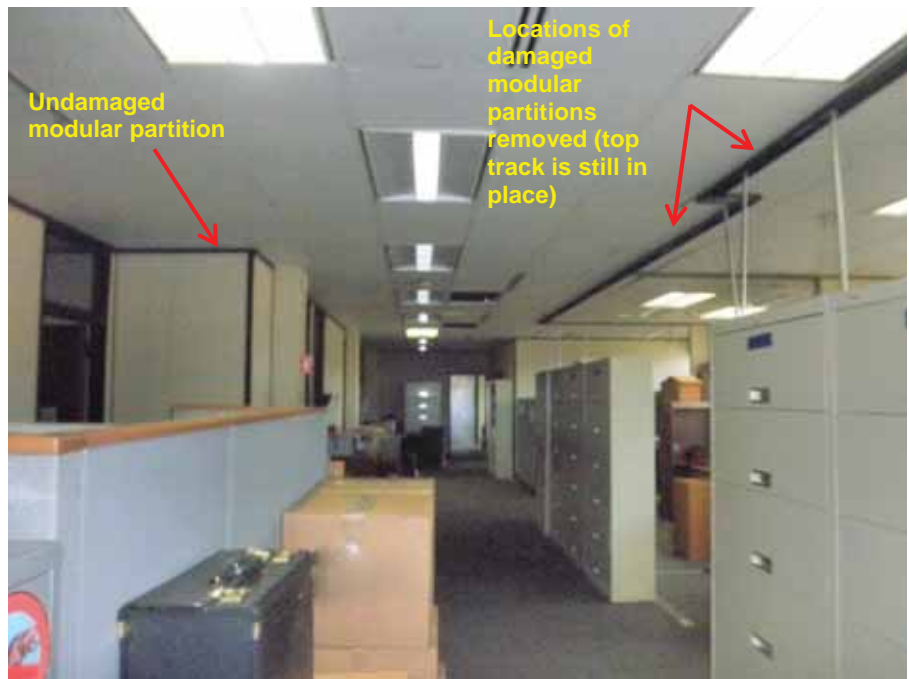
Figure 4-35 Third floor of building after the earthquake. Modular partitions similar to those at the left were damaged and removed.
