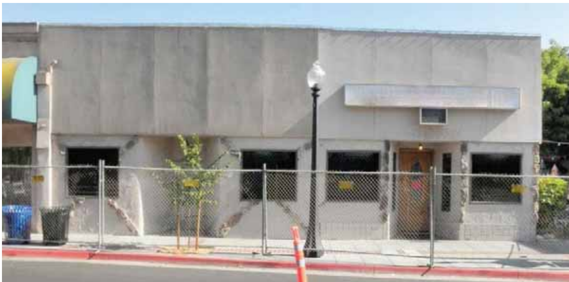
Figure 4-53 Front elevation of Buildings B2/B2A.
