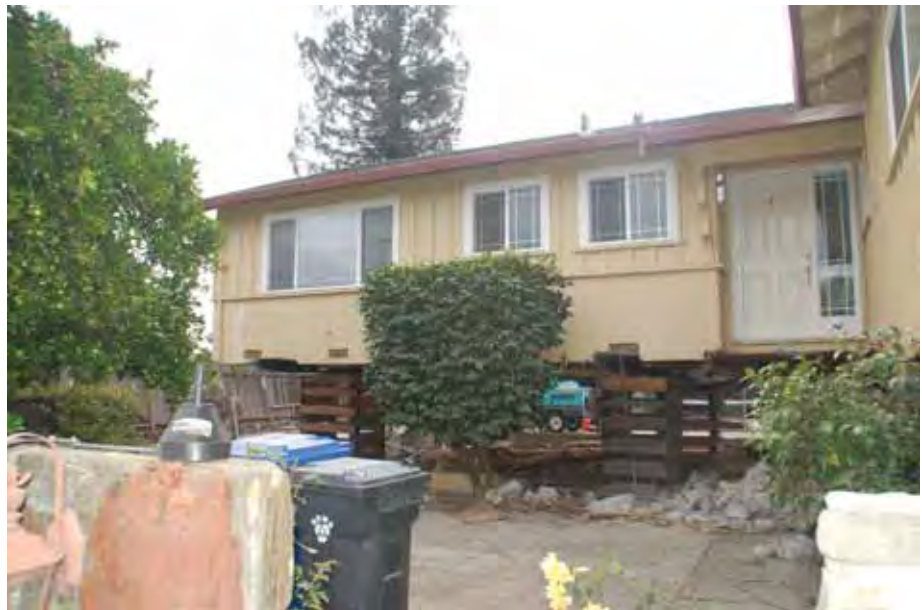
Figure 7-11 Structure raised for foundation repair.
