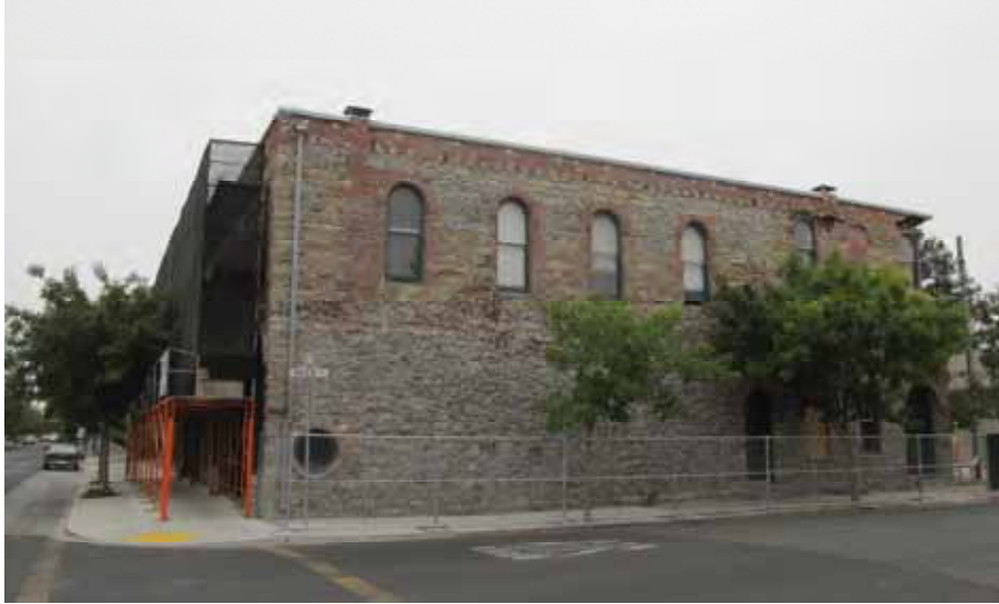
Figure 12-4 Scaffolding used as a barricade on damaged URM building.
