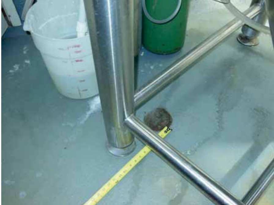
Figure 4-90 Unanchored tank shifted approximately 8 inches.
