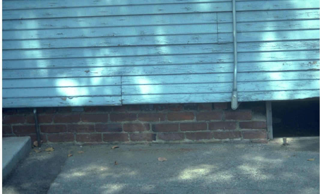
Figure 5-2 Brick masonry foundation wall.
