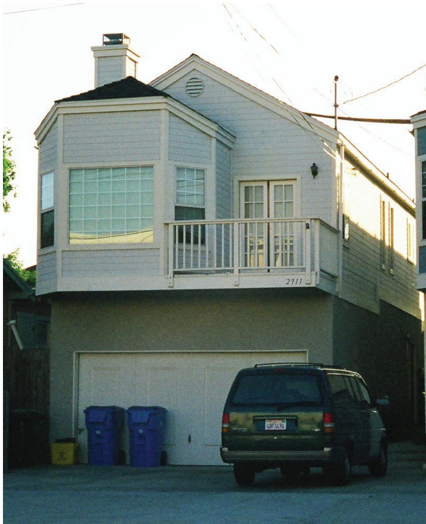
Figure 8-3 House where there appears to be insufficient wall width on each side of the garage door for effective wood structural panel shear wall sheathing (from ATC, 2002).
