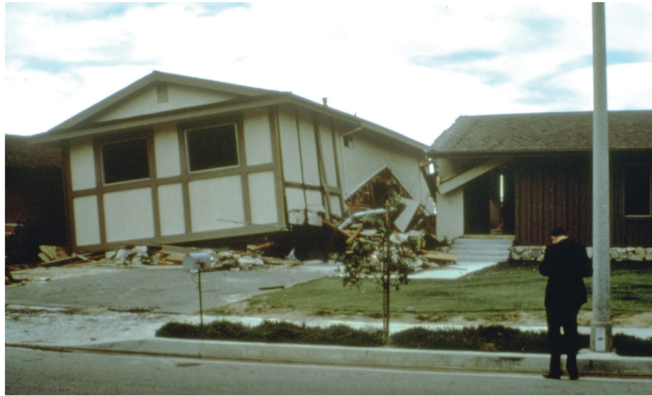
Figure 2-19 Split-level house with damage and collapse at the garage-level walls at two-story portion (from ATC, 2002).
