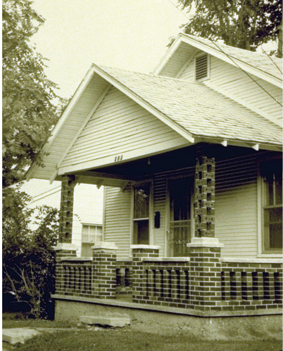
Figure 7-16 Brittle slender masonry porch support posts that will likely collapse during earthquake shaking (from ATC, 2002).
