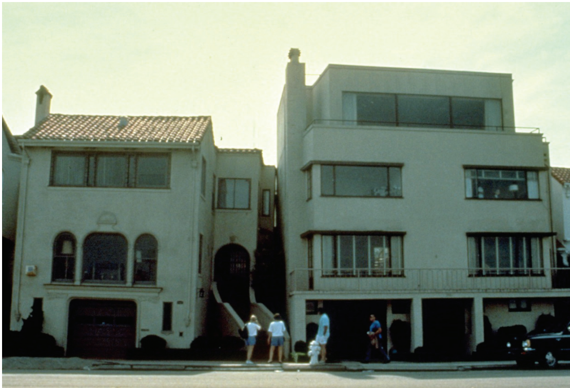
Figure 8-8 Differential settlement of two houses caused by liquefaction along their common property line (from ATC, 2002).
