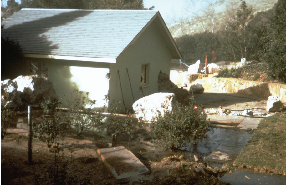
Figure 8-7 Boulder that was shaken loose from the slope above by an earthquake and came to rest against a house (from ATC, 2002).
