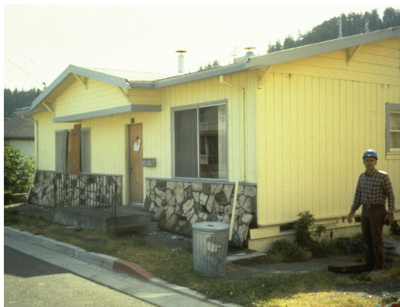
Figure 2-13 Damage to a basement-type house where the sill plate slid on the top of the foundation wall (from ATC, 2002).
