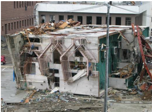
Figure 19. Overturned four story steel building
