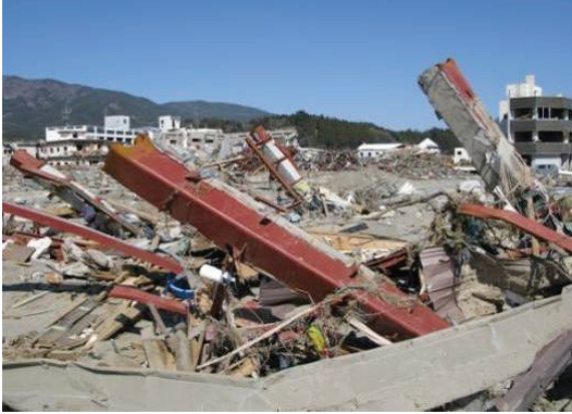
Figure 17. 1 st -story columns falling in the same direction Figure 18. Fracture of the flanges of beams
