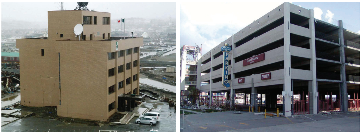
Figure 4: Examples of suitable vertical evacuation structures from Kesennuma, Japan during the Tohoku Tsunami (left) and Biloxi, Mississippi during Hurricane Katrina (right) (FEMA, 2012).
