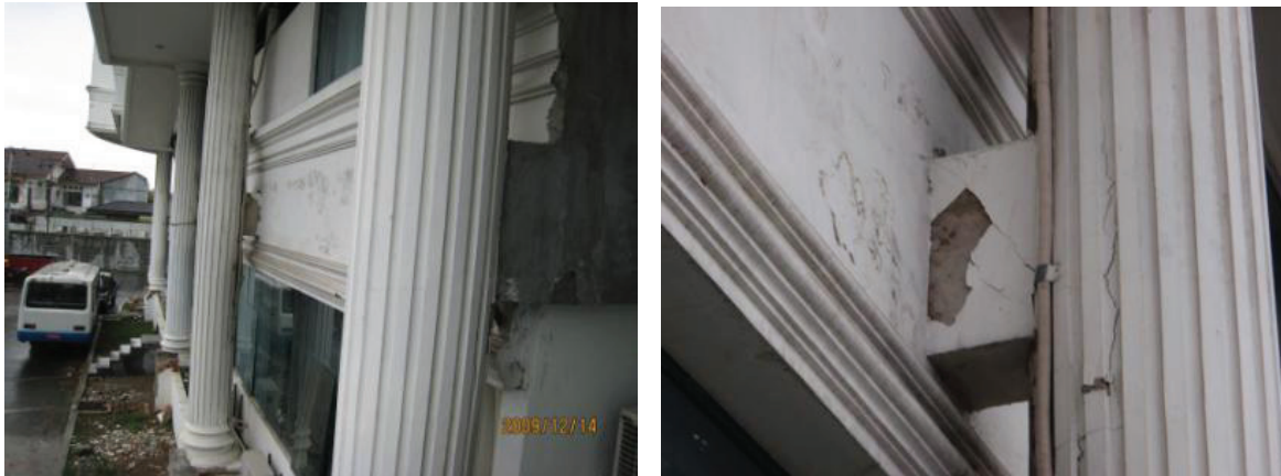
Figure 8. Photograph of Public works office (2)
