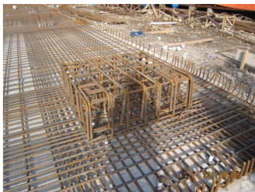
R-bar arrangement of isolator base at 5 May, 2011 R-bar arrangement of mat slab at 6 June, 2011
