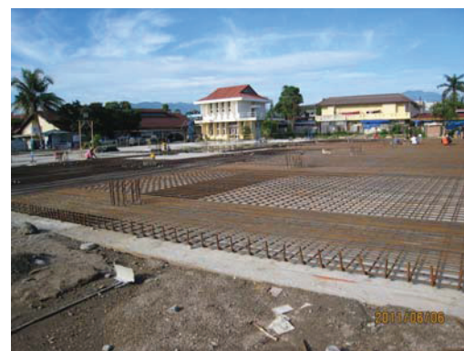
R-bar arrangement of isolator base at 5 May, 2011 R-bar arrangement of mat slab at 6 June, 2011
