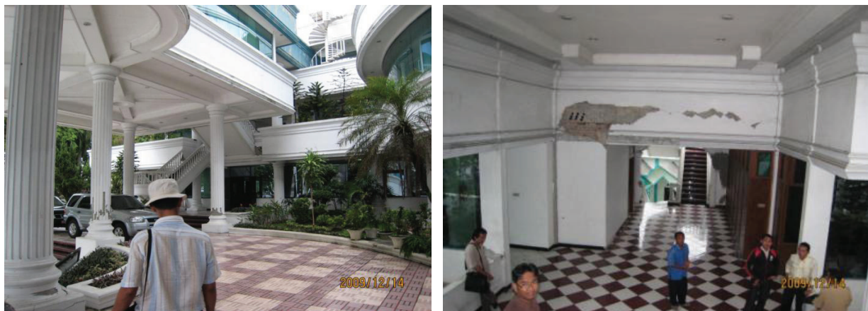
Figure 7. Photograph of Public works office (1)
