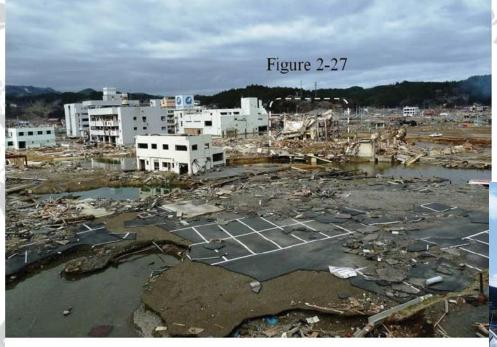
Figure 2-26 Surviving and damaged reinforced concrete buildings in Minamisanriku (photo courtesy of I. Robertson, ASCE, 2012).
