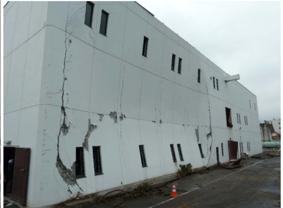
A filtration plant
