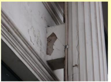
Shear-crack of reinforced concrete beams connected to the outer columns
