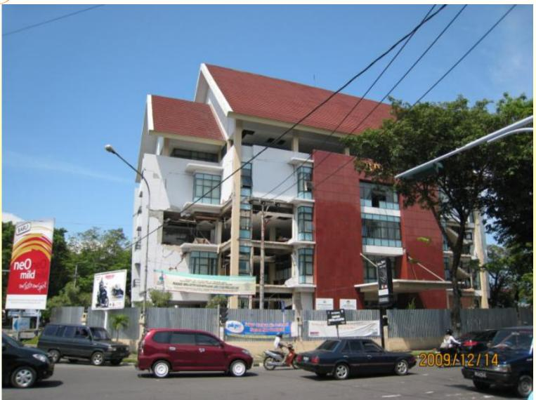
Reinforced concrete rigid frame structure of 6-story with brick wall
