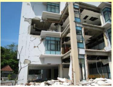
Damage of exterior brick wall and curtain wall
