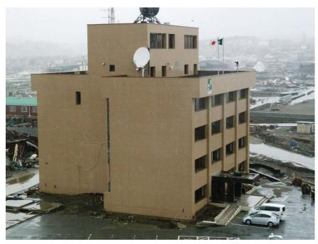
Figure A-1 Successful designated vertical evacuation building in Kesennuma Port, Japan.
