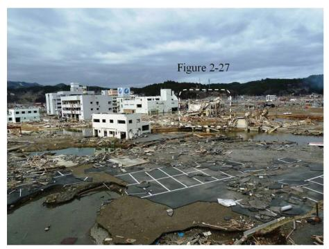
Figure 2-26 Surviving and damaged reinforced concrete buildings in Minamisanriku (photo courtesy of I. Robertson, ASCE, 2012).
