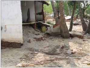
Figure 2-14 Damaged masonry beach house in Devanaanpattinam, India (2004 Indian Ocean Tsunami).
