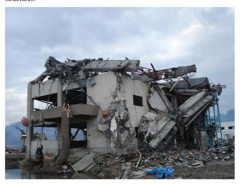
Figure 2-27 Collapsed top floor of reinforced concrete building with steel truss roof (photo courtesy of I. Nistor, ASCE, 2012).
