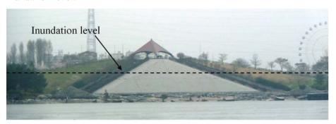
Figure 2-25 Potential evacuation earth mound at West end of Sendai Port (photo courtesy of I. Robertson, ASCE, 2012).
