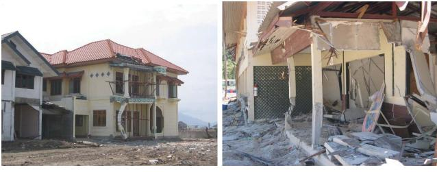
Figure 2-17 Damage to non-engineered concrete columns due to debris impact (photos courtesy of M. Saatcioglu, A. Ghobarah and I. Nistor, CAEE, 2005).
