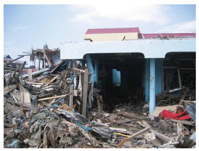
Figure 2-18 Damage to corner column due to debris damming (photo courtesy of M. Saatcioglu, A. Ghobarah and I. Nistor, CAEE, 2005).
