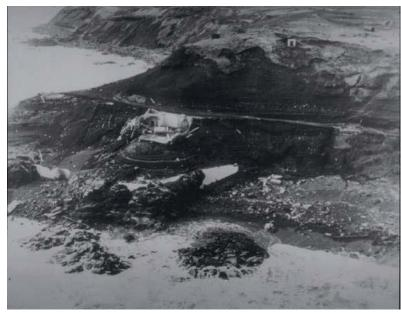
Figure 2-9 Scotch Cap Lighthouse destroyed by the 1946 Aleutian Tsunami.
