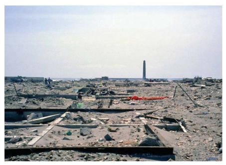
Figure 2-10 Total destruction of a group of wood-frame houses in Aonae Village, Okushiri Island, Japan (1993 Okushiri Tsunami).
