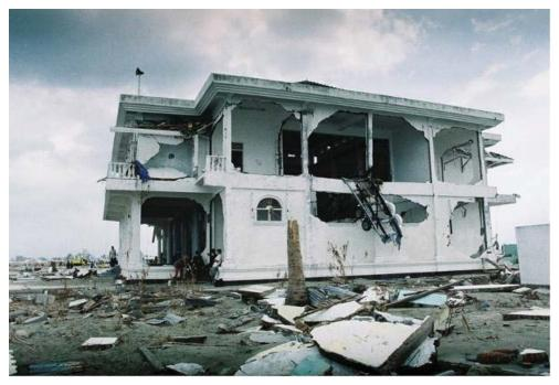
Figure 2-15 Example of surviving reinforced concrete mosque in Uleele, Banda Aceh (photo courtesy J. Borerro).
