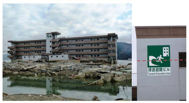
Figure 2-23 Minamisanriku designated coastal evacuation building – note tsunami trace on sign (photo courtesy of I. Robertson, ASCE, 2012).
