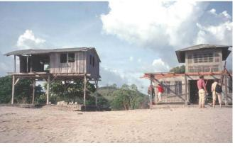
Figure 2-11 Beach houses with varying levels of damage in El Popoyo, Nicaragua (1992 Nicaragua Tsunami). All three houses are in the same vicinity.
