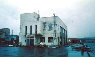
Figure 2-13 Examples of reinforced concrete structures that survived the 1993 Okushiri Tsunami: vista house at Cape Inaho (left); and fish market in Aonae (right) (photo courtesy N. Shuto).
