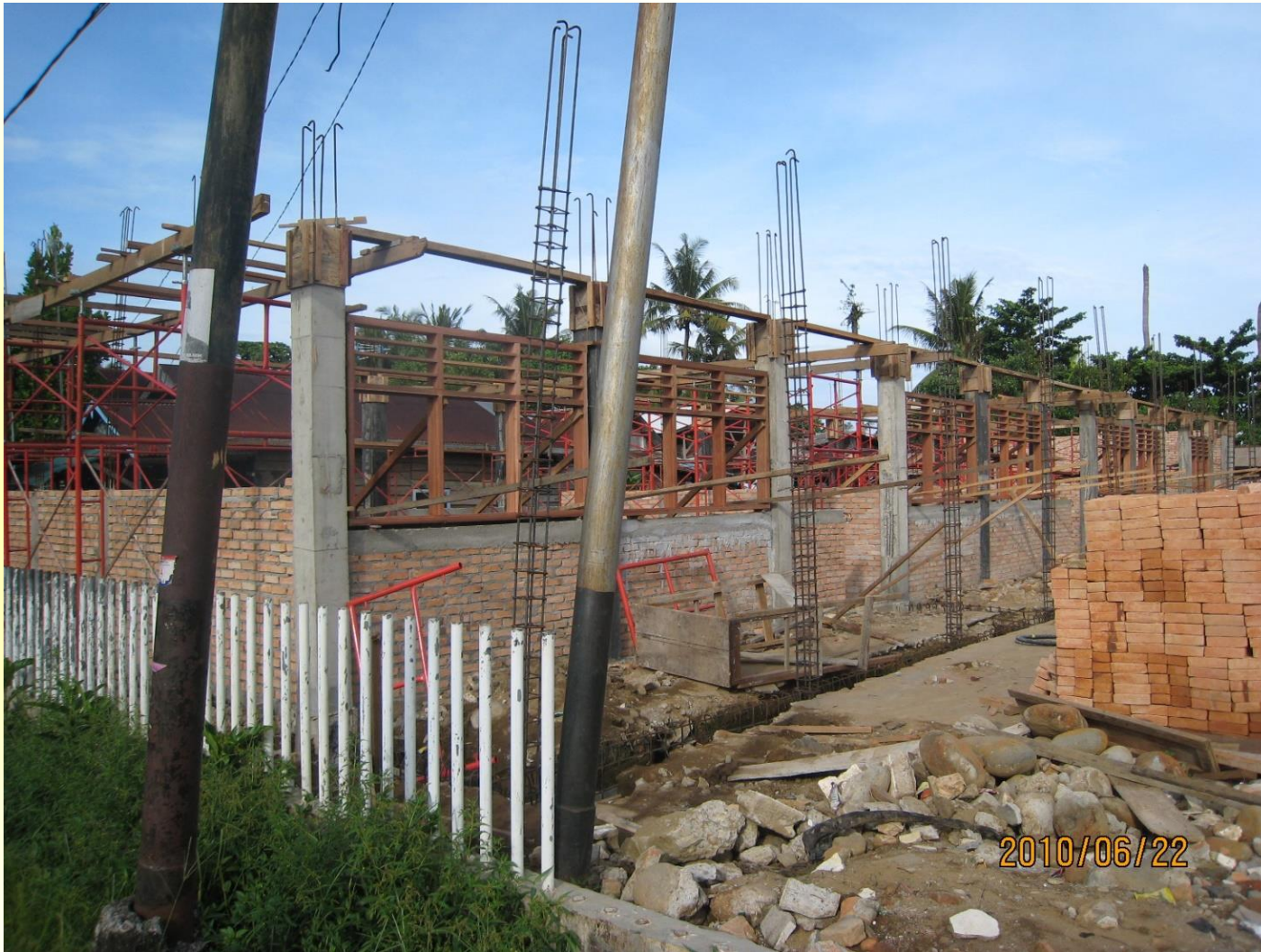
Reinforced concrete column/beam with non-structural brick wall
