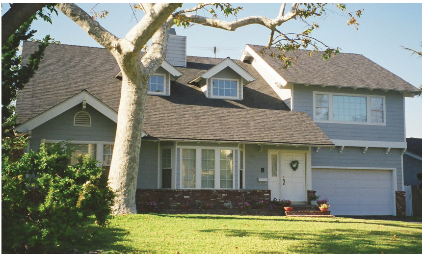
Figure C-14 Split-level house, where the section of flooring above the garage is at a lower level than the main second-floor level (from ATC, 2002a).
