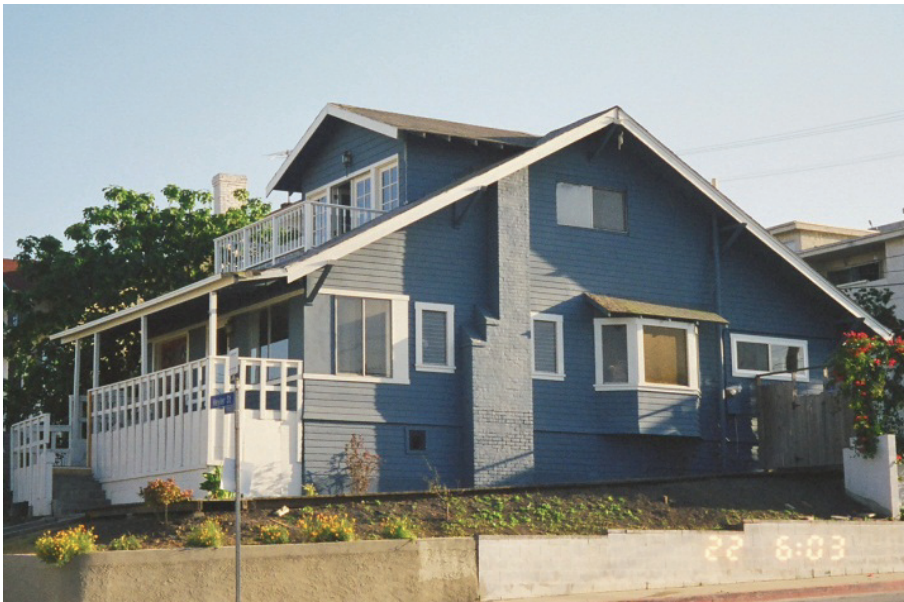
Figure C-3 Typical older one and one-half-story cripple-wall crawl-space house (from ATC, 2002a).
