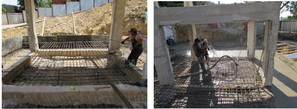
*Figure 3. Stages of strengthening of foundation of test building.*
