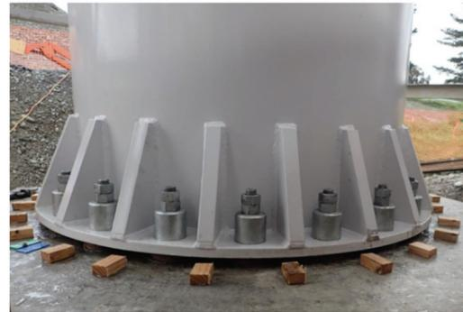
*Figure 6. Construction of Wigram-Magdala Bridge pier with low damage joints.*
