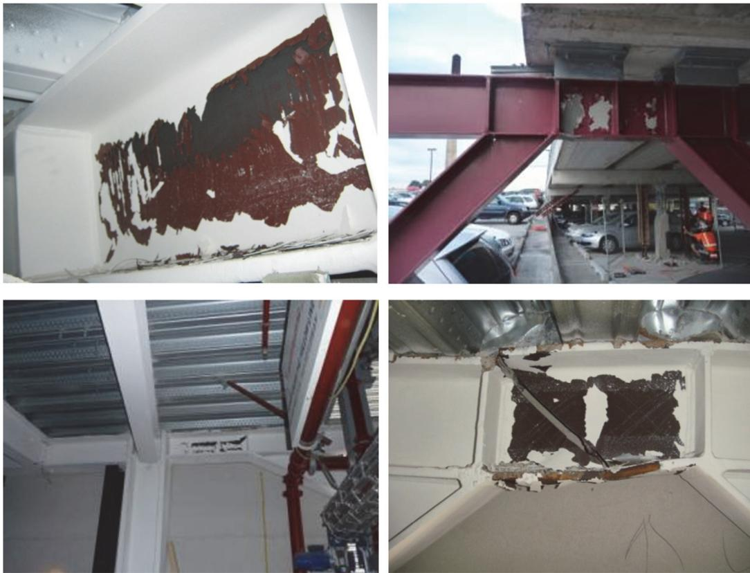
Figure 2. Yielded active links from Christchurch 22/02/2011 Earthquake (from (Clifton, Bruneau et al. 2011). Clockwise from top left: (a) Yielded active link level 3, 12 storey HSBC Tower, (b) Active link at edge of building with slight flange local buckle, level 1, 3 storey car parking building; (c) Fractured and yielded active link, level 6, 22 storey Pacific Tower; (d) Yielded active link, level 4, 22 storey Pacific Tower.
