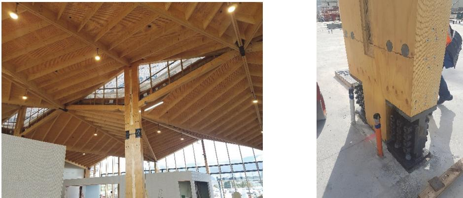
*Figure 8. Internal view during construction and detail of RSFJ.*
