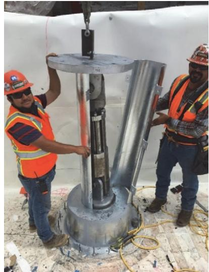
b) Photograph of the damper being installed at the construction site.
