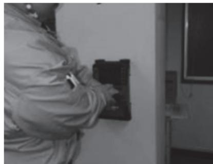
*Photo 4. Investigation of re-bar arrangement by non-destructive test.*
