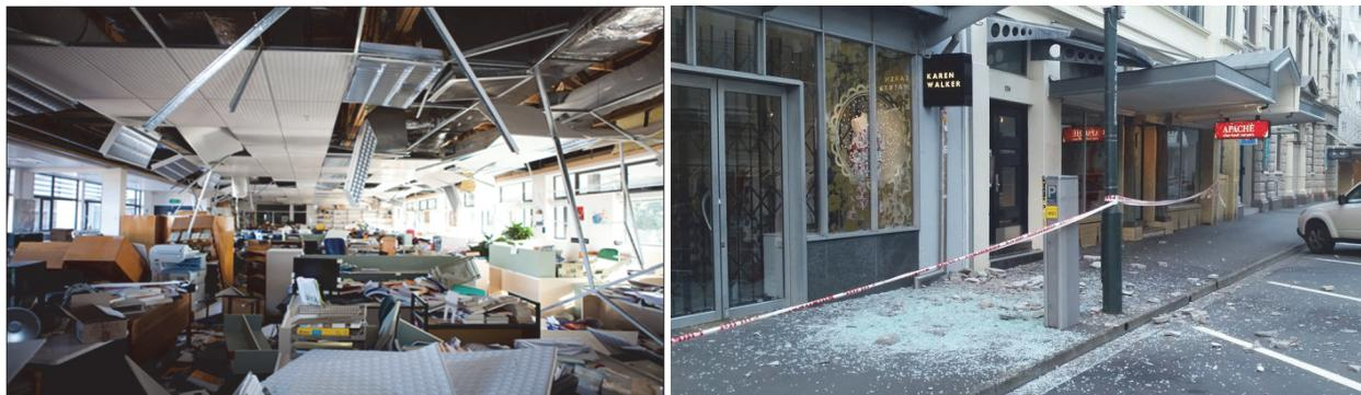
*Figure 1: Illustrating damage to non-structural elements observed in the Canterbury earthquakes (left, from Dhakal, 2010) and Kaikoura earthquake (right, from Radio NZ/Susie Ferguson).*
