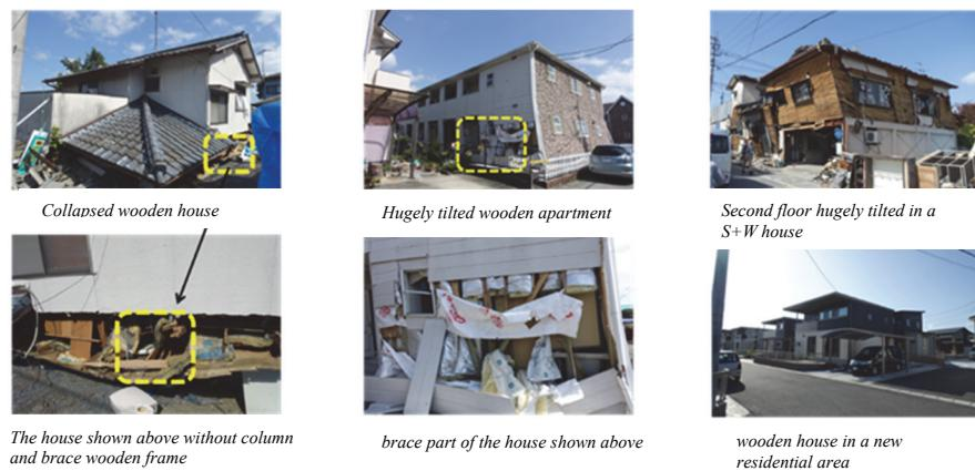
Photo 5. Examples of damage to wooden houses affected by the Kumamoto Earthquake.
