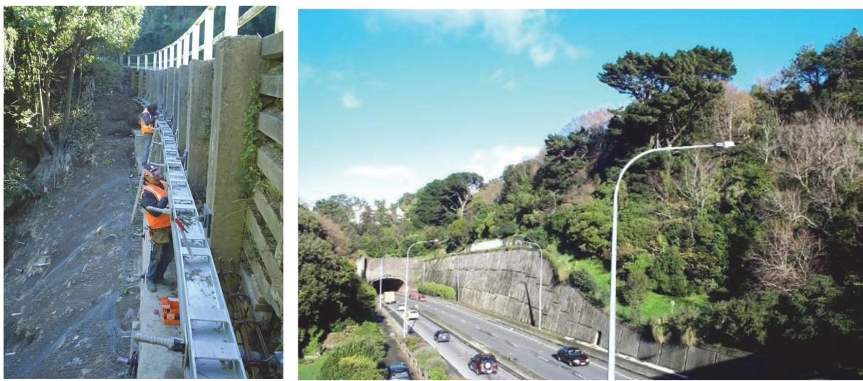
Figure 1. Strengthening of Ngaio Gorge retaining walls (left), Terrace tunnel approach walls (right).
