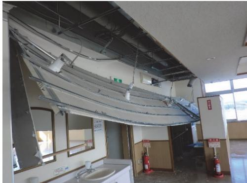
Figure 1. Damage of ceilings
