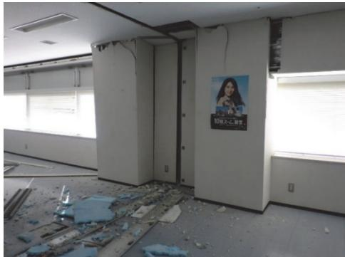
Figure 5. Damage of expansion joints.
