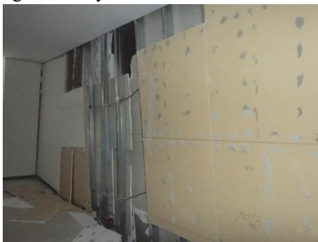
Figure 3. Damage of dry partition.
