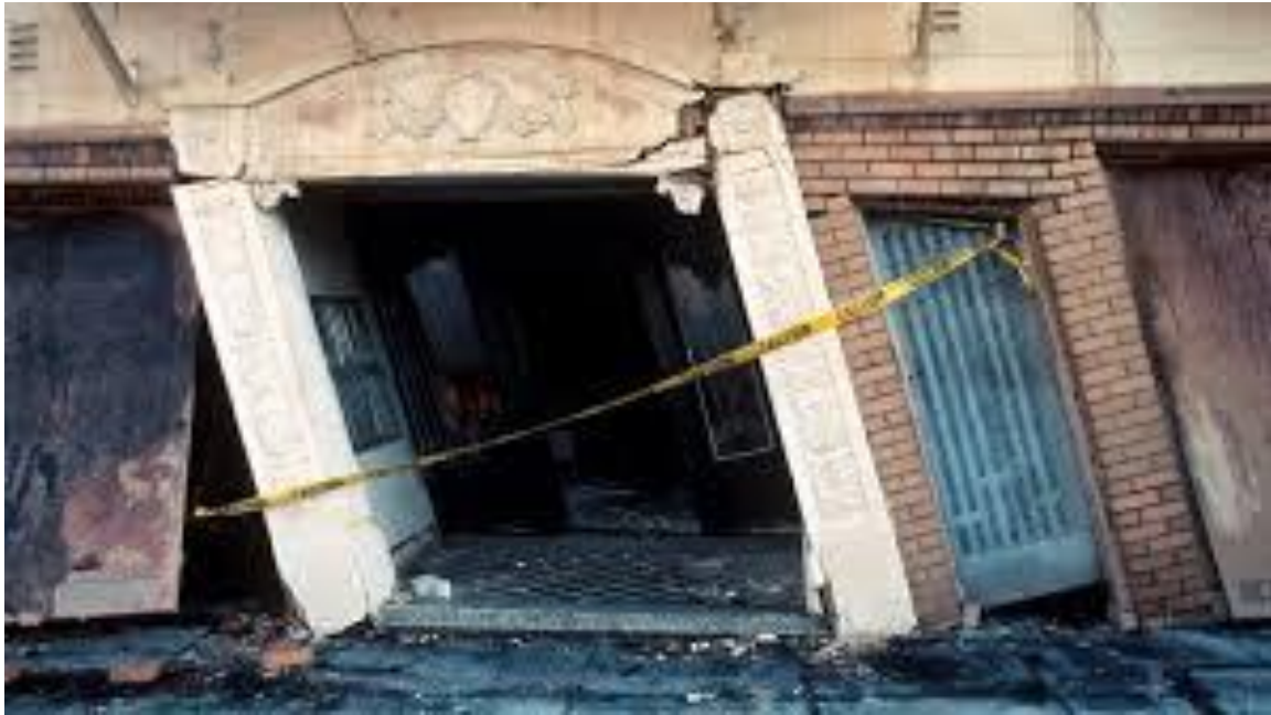
Figure 2-11 – Soft story racking damage.
