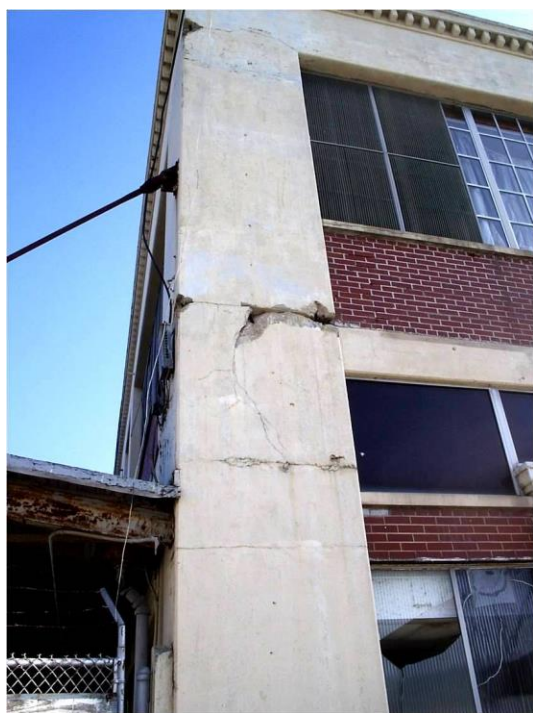
Figure 3-1 - Damaged concrete column, 2005 Hurricane Katrina
