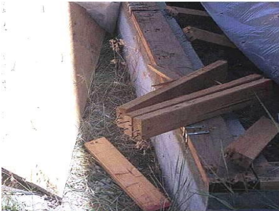
Figure 4-20 – House with cripple wall failure, 1992 Big Bear Earthquake
