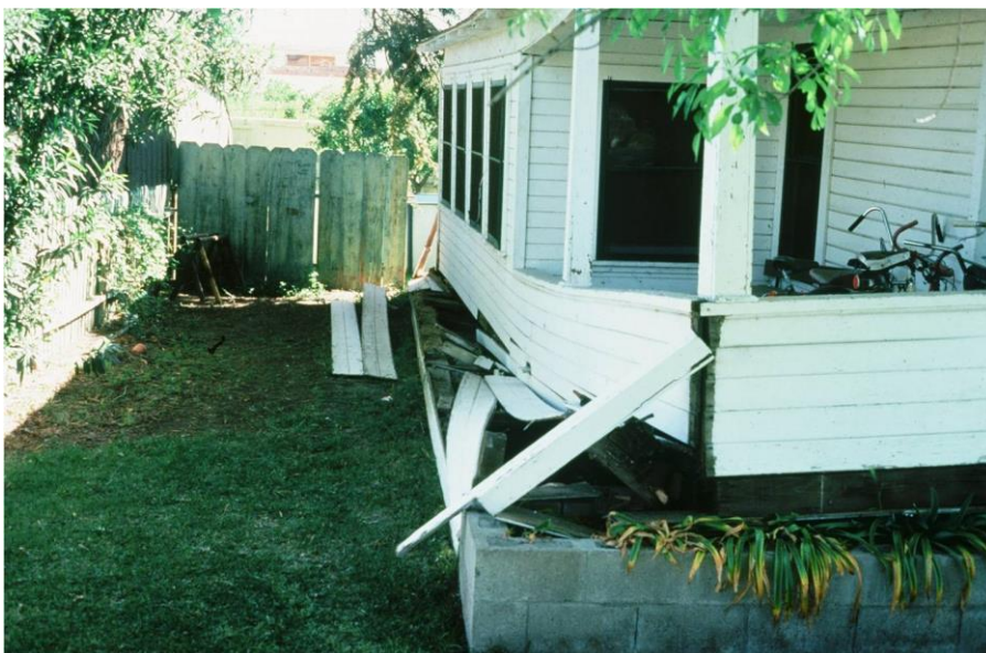
Figure 2-4 – House off of its foundation
