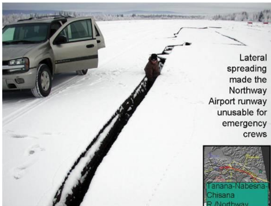
Figure 6-9 – Airport runway with lateral spreading, 2008 Denali Earthquake, Alaska
