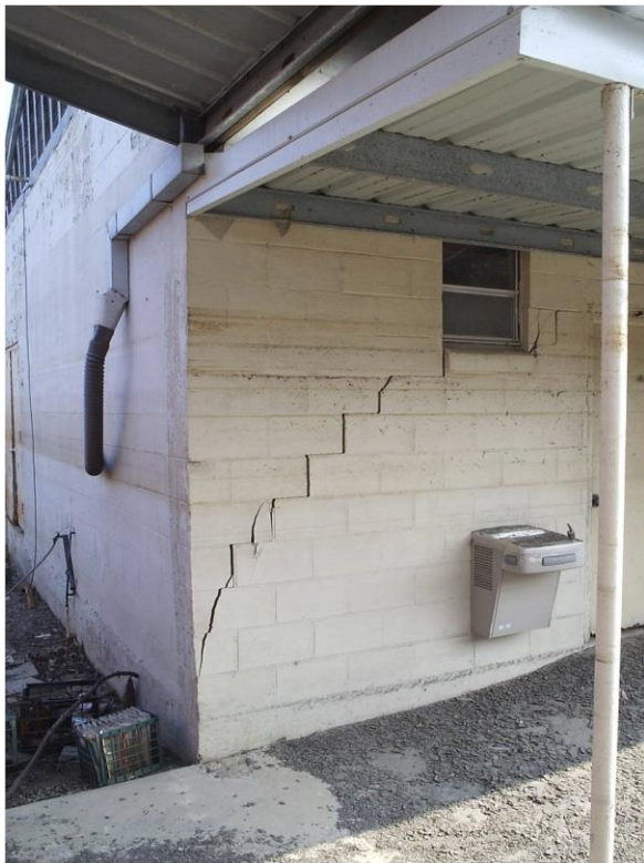
Figure 3-16 – Unsafe house due to cliff erosion, Pacifica, CA, 1998 El Nino Storms
