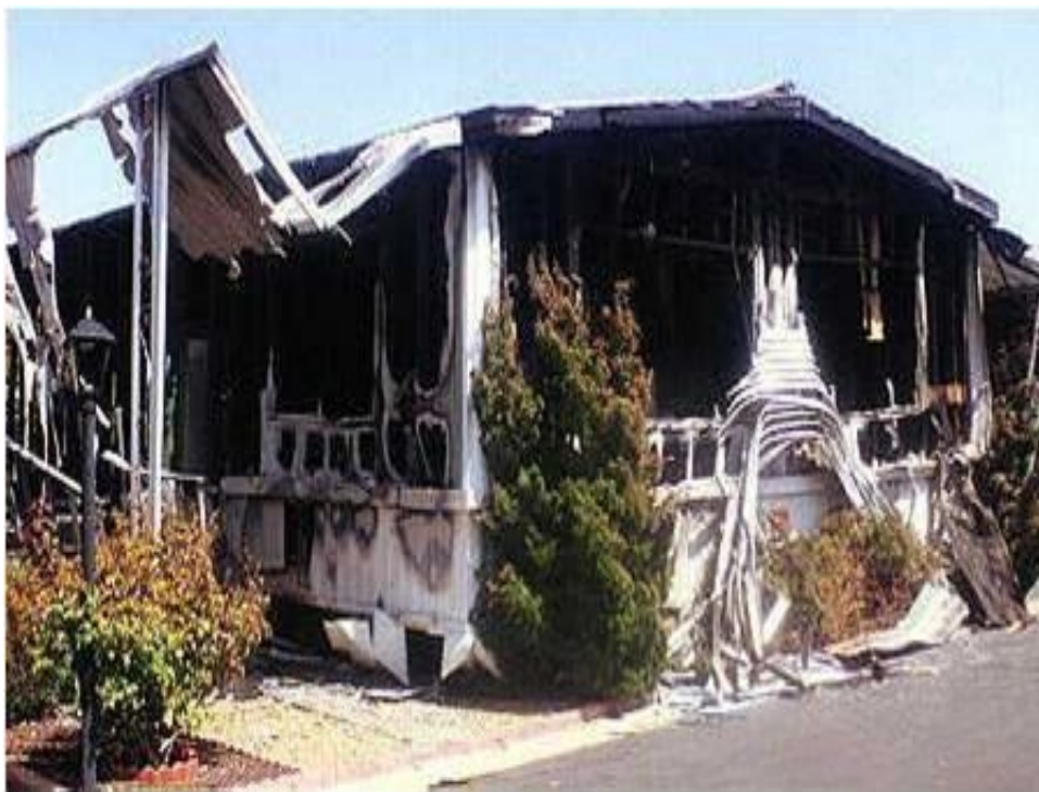
Figure 4-3 – Mobile home partially fallen, 1992 Landers/Big Bear Earthquakes
