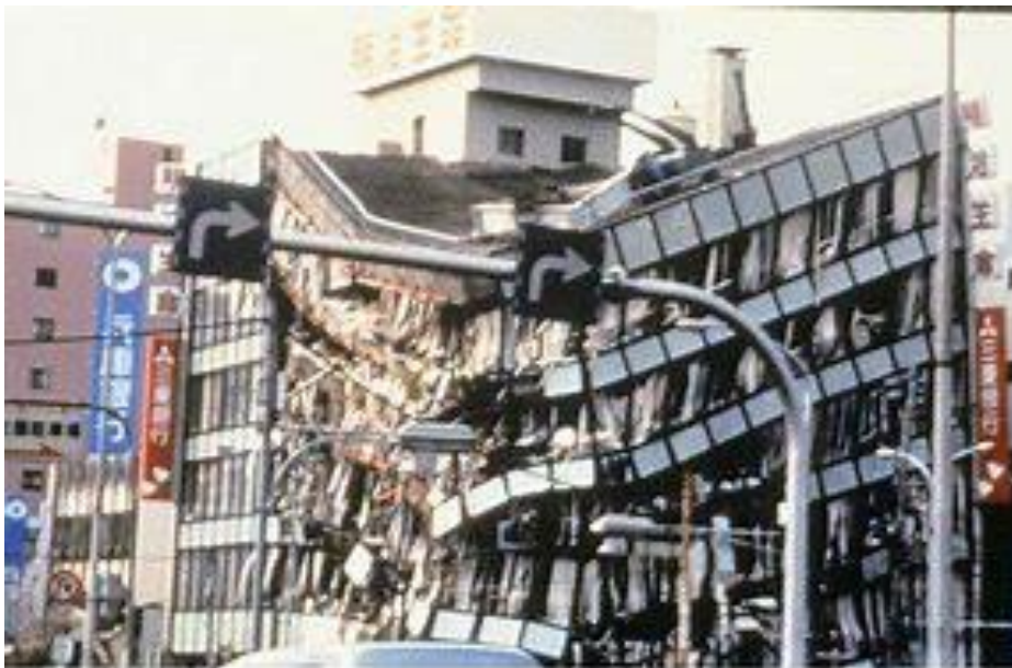
Figure 2-10 – Partial collapse of structure.
