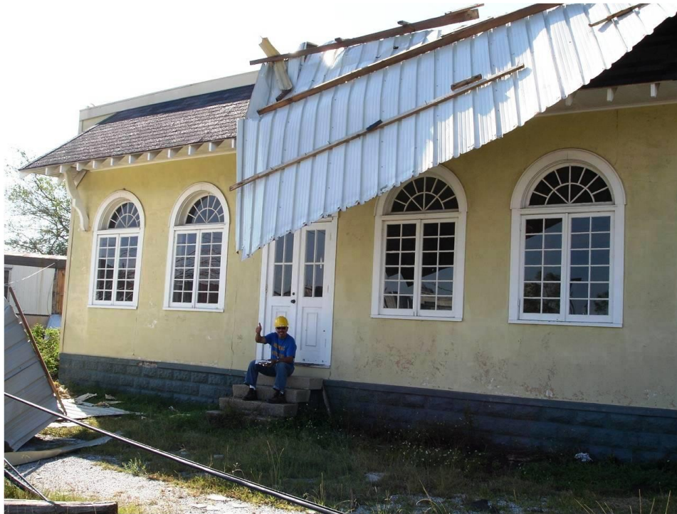
Figure 7-5 – Roof fragment falling hazard, 2005 Hurricane Katrina
