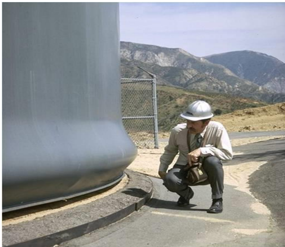
Figure 6-21 – Steel water tank with ‘elephant’s foot’ buckling
