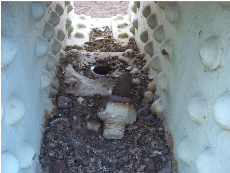
Figure 2-25 – Damage to water tower concrete footing
