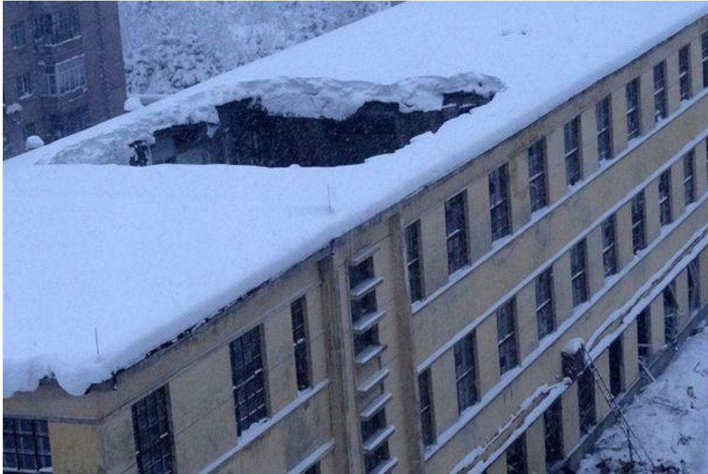
Figure 3-34 - Roof collapse due to snow
