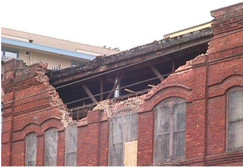
Figure 2-16 – Unreinforced masonry wall failure, 2001 Nisqually Earthquake.
