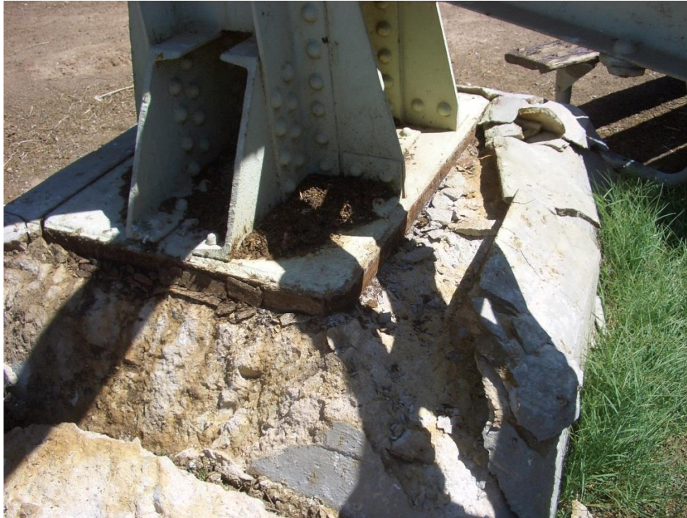
Figure 2-25 – Damage to water tower concrete footing
