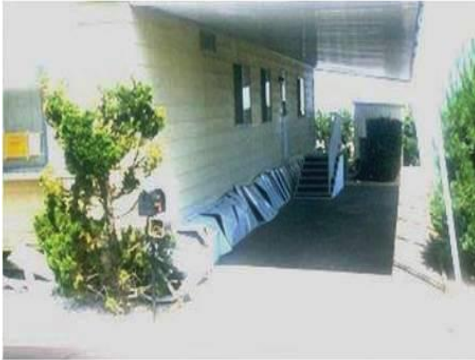
Figure 4-3 – Mobile home partially fallen, 1992 Landers/Big Bear Earthquakes
