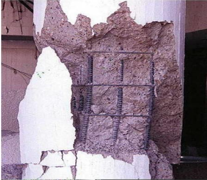
Figure 2-20 – Detail of damaged column showing P-delta effect
