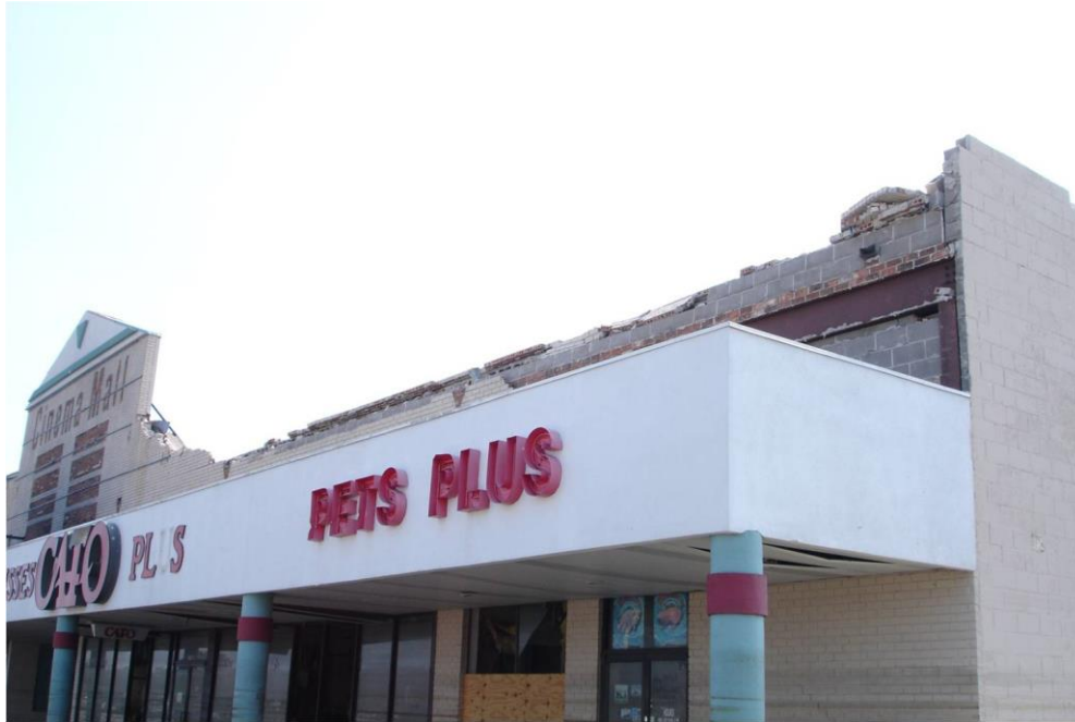
Figure 3-2 – Parapet blown off, 2005 Hurricane Katrina
