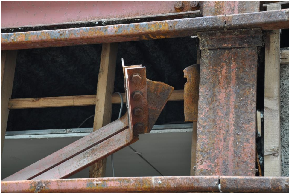
Figure 2-20 – Detail of damaged column showing P-delta effect
