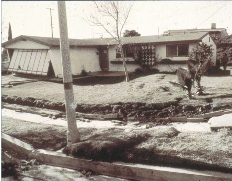
Figure 6-2 – Surface rupture, 1971 Sylmar Earthquake
