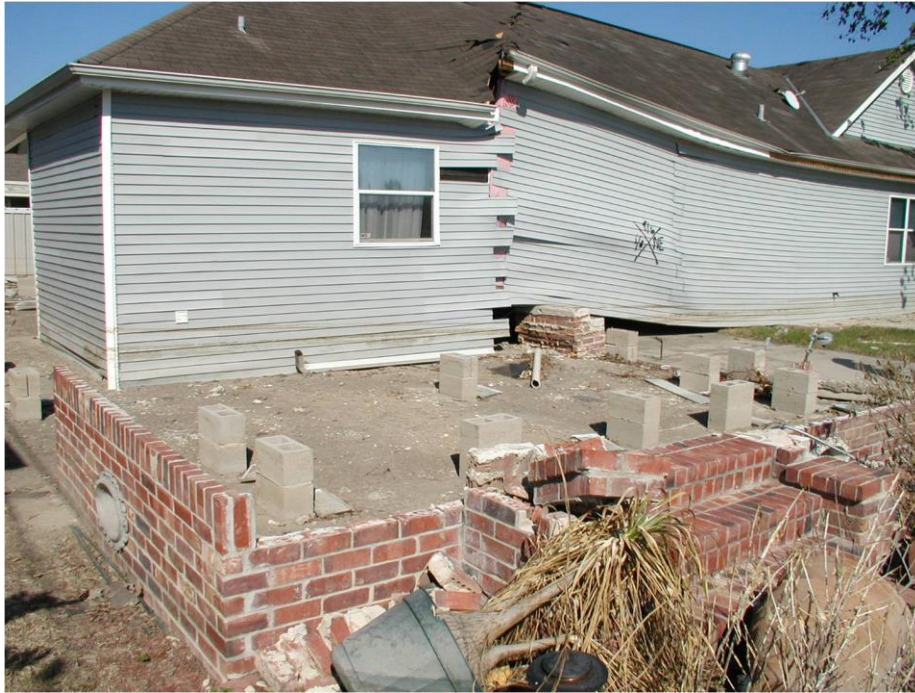
Figure 3-19 – Wood frame home floated off its foundation, 2005 Hurricane Katrina
