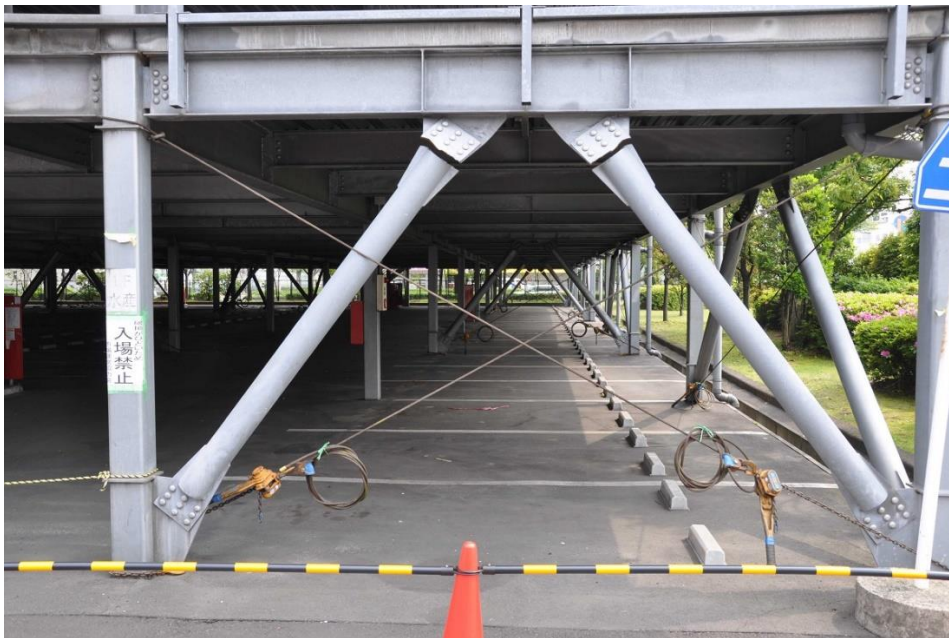
Figure 2-23 – Failed gusset plates on lateral bracing
