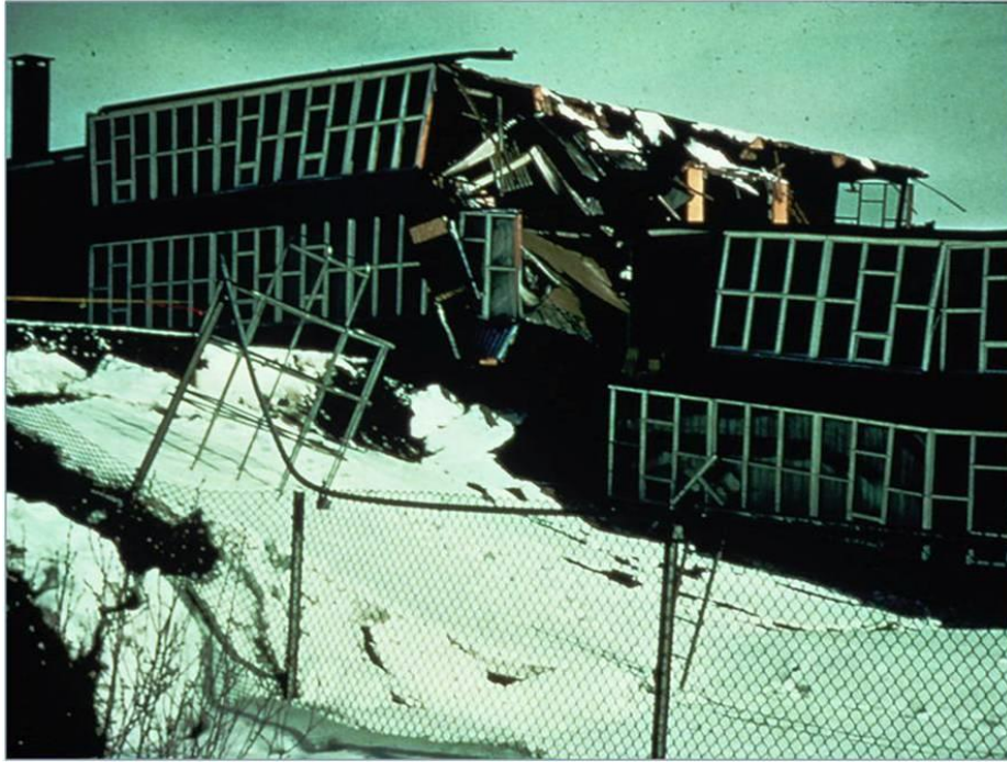
Figure 2-9 – Ground scarp through building
