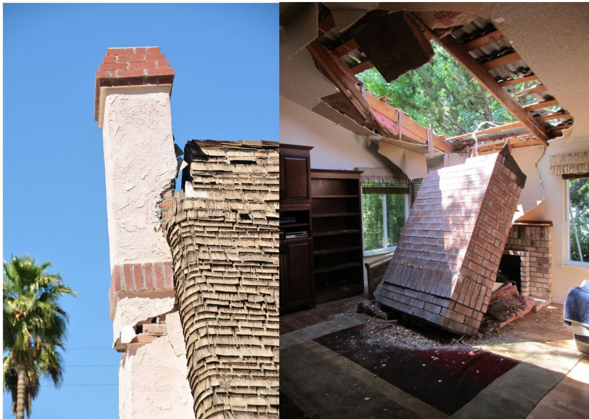
Figure 2-12 – Damaged chimneys
