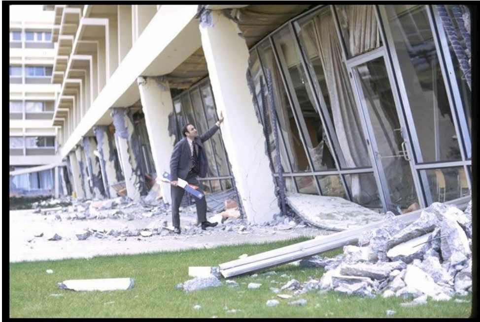
Figure 2-22 – Failure of concrete moment frame.
