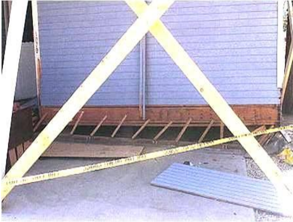
Figure 4-20 – House with cripple wall failure, 1992 Big Bear Earthquake
