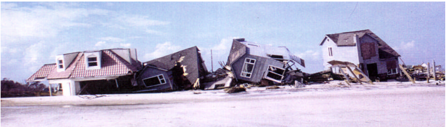
Photo shows the type of wave-action damage sustained by homes at the ocean's edge. R. Dean photo.
