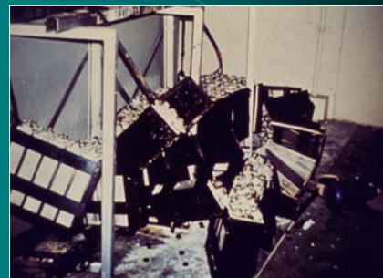
Acid Spill from Cracked Batteries
