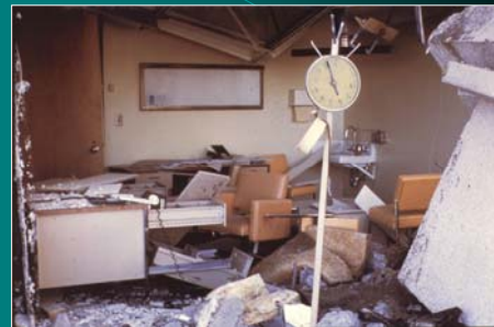
Olive View Hospital 1971 San Fernando Earthquake
