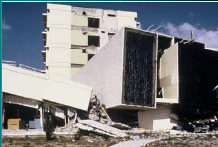
Olive View Hospital 1971 San Fernando Earthquake
