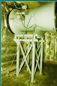
Olive View Hospital 1994 Northridge
