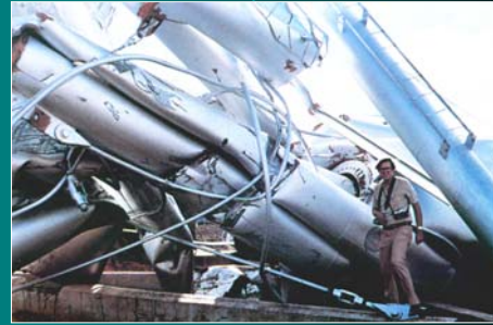
Collapsed Water Tower - Brawley, California
