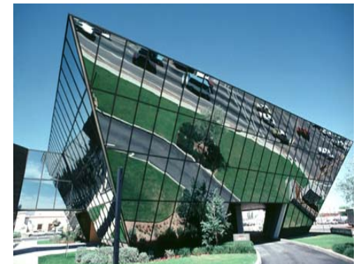
An unusually shaped building for which the applicability of any of the ASCE 7 Analytical Methods is questionable (from SEAW/ATC-60 Commentary on Wind Code Provisions ).
