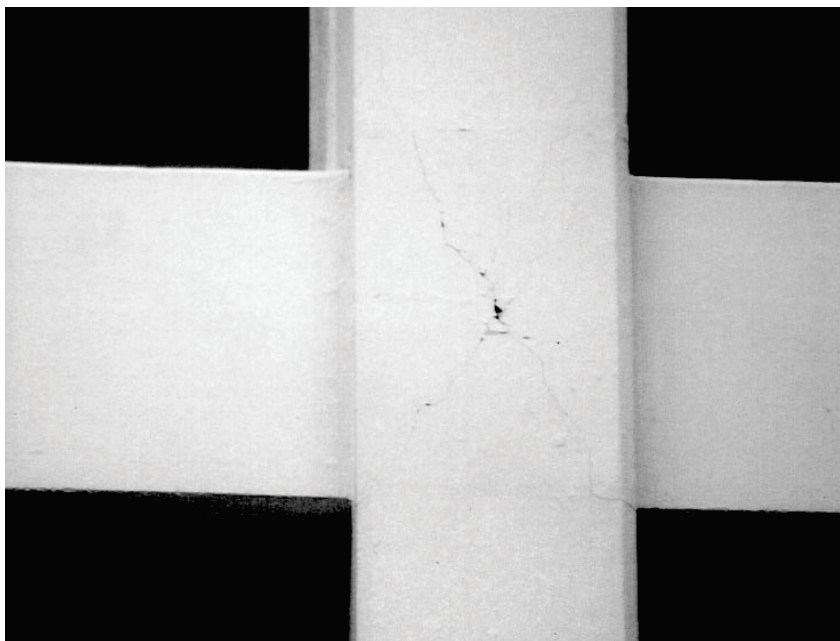
Figure 7-16 Shear distress in beam-column joint (Trifunac et al., 1999).
