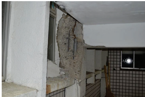
(c) Extensive damage to Column E8
