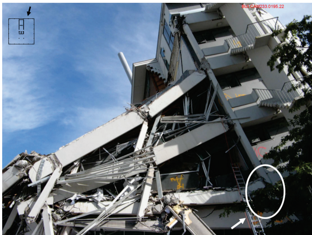
Figure 8-11 Photo showing overview of collapsed building from north; circle indicates location of axial failure of east wall (obscured; adapted from Jury and Sharpe [2011]).
