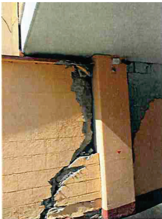
Figure 10-17 Damage to first story masonry walls in north building boundary (Dirac Ingenieros Consultores, 2019b).
