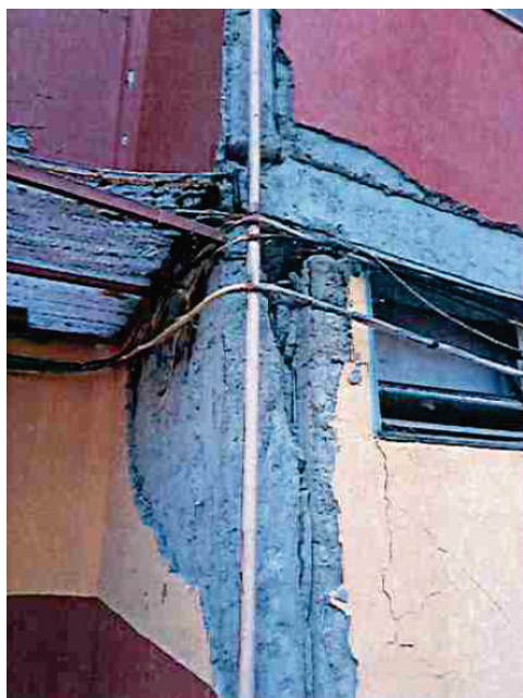
Figure 10-14 Damage at the edge of first story structural wall (Dirac Ingenieros Consultores, 2019b).
