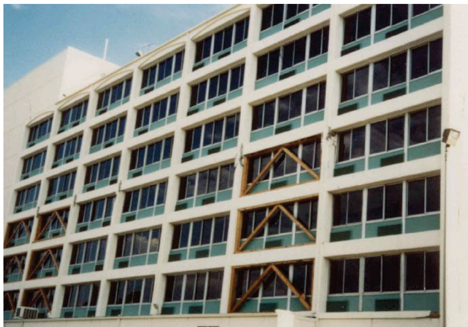
Figure 7-12 Structural damage to columns of south exterior frame after 1994 Northridge Earthquake (Concrete Coalition, 2019). Braced frames added after the earthquake as temporary lateral support.
