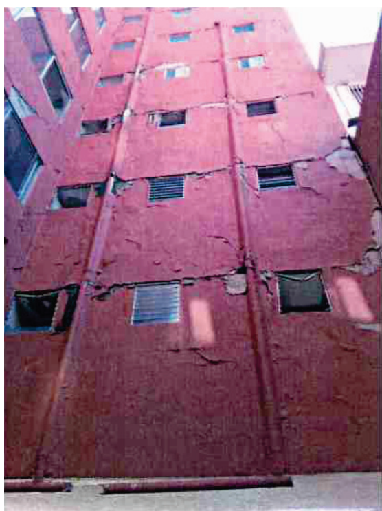
Figure 10-16 Damage to façade masonry walls in north illumination shaft (Dirac Ingenieros Consultores, 2019b).
