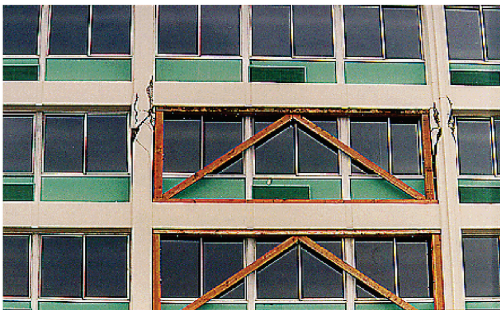
Figure 7-13 Structural damage to fifth floor columns of south exterior frame after 1994 Northridge Earthquake (Naeim et al., 2005). Braced frames added after the earthquake as temporary lateral support.
