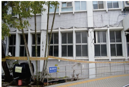
(a) Column damage in Frame A
