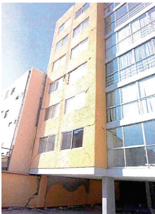
Figure 10-18 Photograph showing damage to first story masonry walls and close proximity of adjacent building in south boundary (Dirac Ingenieros Consultores, 2019b).
