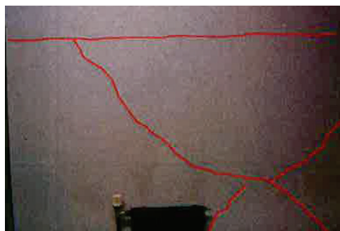
(c) Cracking ( \leq 0.2 mm)
