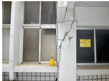
(b) Column damage (typical)
