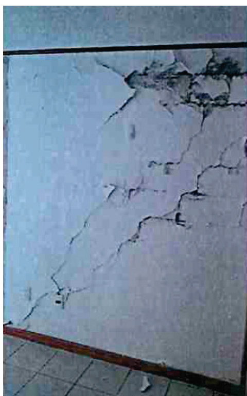
Figure 10-20 Damage to interior masonry walls in apartment unit (Dirac Ingenieros Consultores, 2019b).
