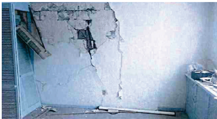
Figure 10-19 Damage to interior masonry walls in apartment unit (Dirac Ingenieros Consultores, 2019b).
