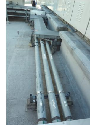
Some of the equipment on the roof of the six-story main building, none of which was damaged in the earthquake. Our investigation revealed good design details for the anchorages and braces of the equipment, piping, and other systems.
