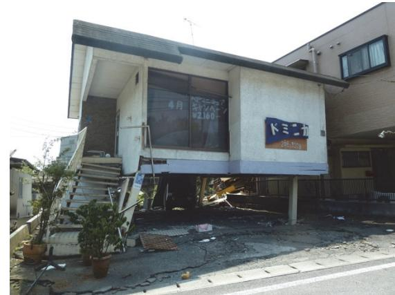
On the left is a practically undamaged house, which is not far away from the severely damaged house on the right. The difference in performance is primarily due to lack of bracing in the garage in the house on the right. Note the unbroken window on the second floor.
