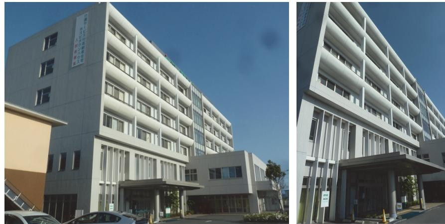
The main building of the hospital was built in 2012 and showed no visible structural damage. The only significant damage inside the building was minor spalling at seismic (expansion) joints. There was also minor settlement of the ground and of excavation backfills around the buildings.
