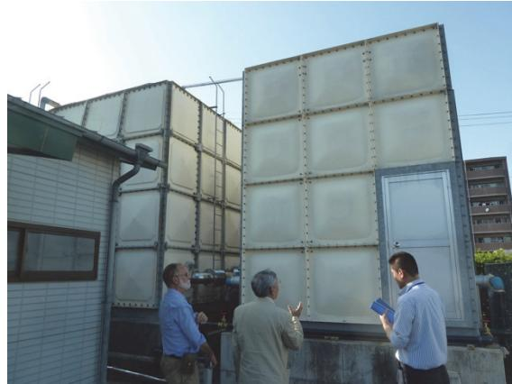
**Two anchored potable water tanks lost content when the rigid piping that interconnected them failed due to differential tank movement during the earthquake. The repaired lines are shown on the left. A flexible pipe connection between them would have prevented the only significant equipment and systems damage at the hospital.**
