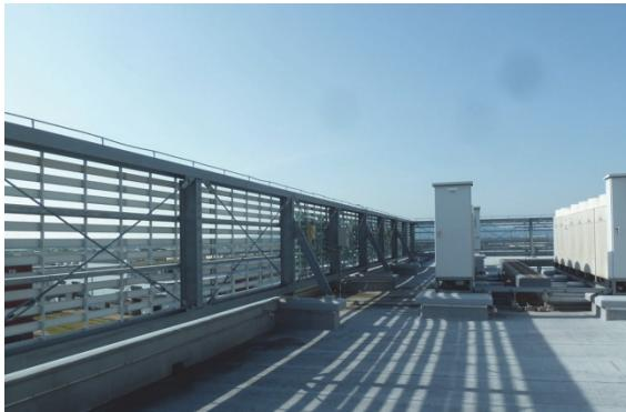
A partial view of one of the two-story hospital buildings (left) and the undamaged steel framed and braced parapet on the roof of the 6-story main building.
