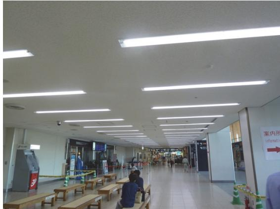
The rigid suspended ceilings throughout the new terminal performed well. We did not notice any significant damage. There was minor damage at interfaces with columns and walls. In the past, damage to flexible suspended ceilings at airports has been a major cause of service interruptions.
