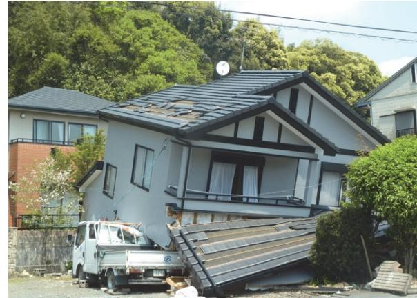
**Another house with too many openings (windows) and not enough walls on the ground floor. Note the relatively undamaged houses behind and on the right of the collapsed house.**
