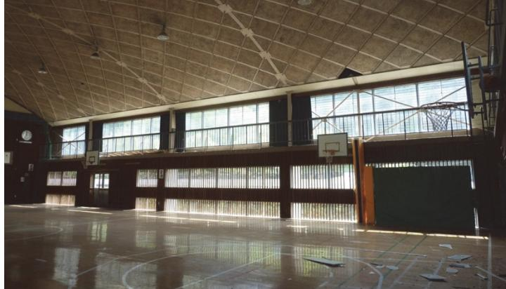
**Interior of the virtually undamaged gym. A few lightweight ceiling tiles fell because of inadequate attachment to the structural roof (and ceiling). The debris can be seen in the lower right corner. Note that all of the windows are intact.**
