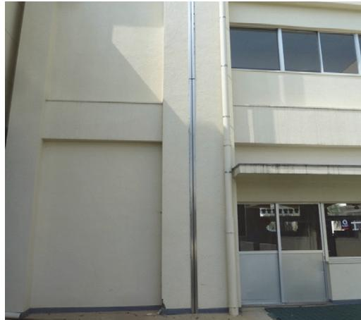
Another obvious strengthening detail - note that the two story solid concrete wall has been added to strengthen the original school. It replaced the windows that were there in the original design. This "shear wall," which adds strength, is a common retrofit detail and works well for this type of concrete-frame construction.
