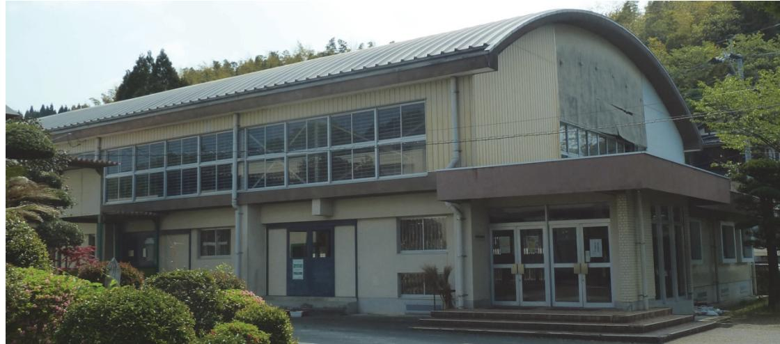
The Tsumori Elementary School gym. One quick look at the building, and adequate familiarity with school earthquake strengthening programs in Japan and around the world, was sufficient for me to realize that this school had been strengthened for earthquakes after it was originally built (well before the more recent earthquake code standards). The steel X-braces (behind the second floor windows and inside the gym) are used often in Japan and elsewhere for strengthening.
