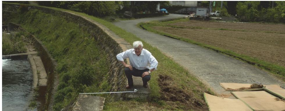
Along the Futagawa fault through a hilly residential area of Mashiki. Here the fault has offset a retaining wall by about 4 feet (1.2m). Houses right on top of the fault were typically completely destroyed. Nearby wood frame houses, not directly on the fault, had various degrees of structural damage – from light to extreme, including many collapses.
