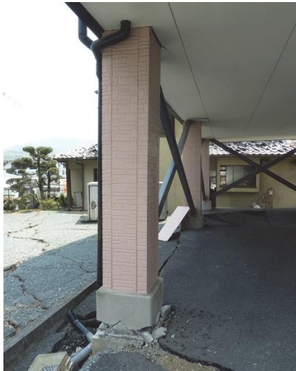
**Damage to a house in the hills above Mashiki primarily caused by local ground failure, either due to minor landsliding or inadequate compaction of fill in the construction of a level building site. The building is leaning to the right; the main ground movement was to the left and downhill.**
