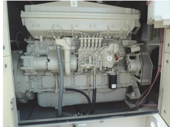
The emergency diesel, located on the roof of the six-story main building, started up upon loss of off-site power. The diesel, plus a second generator in another building, provided adequate power to the hospital following the earthquake until off-site power was restored.
