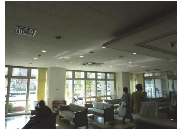
The most obvious and inconsequential damage to the hospital was minor settlement around the periphery of buildings. The photo in the upper left shows some settlement at the main entrance to the hospital. The other three photos are of interiors of the main building, including the lobby (lower right). Note that the undamaged ceilings are rigid, unlike flexible suspended ceilings that are typically easily damaged.
