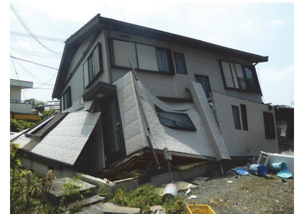
**Other severely damaged houses in Mashiki. Most of the damage that occurred was due to inadequate strength in the lower floor walls, including too many windows. That additional strength can be easily provided by adding bracing with a few more well-nailed plywood sheets.**
