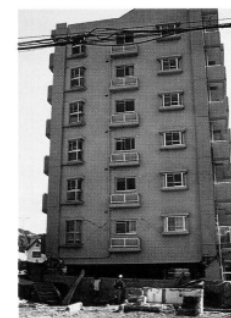
Fig. 12. A post-1981 apartment building that collapsed at the soft first story.
