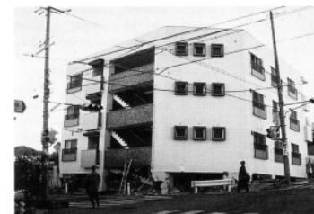
Fig. 10. A pre-1981 apartment building that collapsed at the soft first story.
