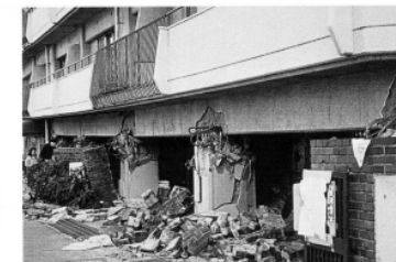
Fig. 11. A pre-1981 apartment building that collapsed at the soft first story.
