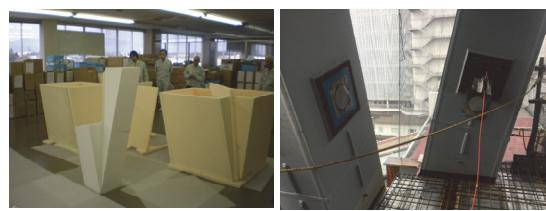
Figure 15. Full-size model and view of concrete filling (3rd to 5th floor branched columns)
