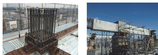
Figure 14. Position of column switching on the 6th floor and erection of 7th floor PCa beams
