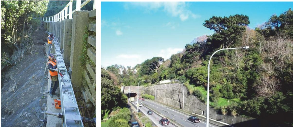
Figure 1. Strengthening of Ngaio Gorge retaining walls (left), Terrace tunnel approach walls (right).
