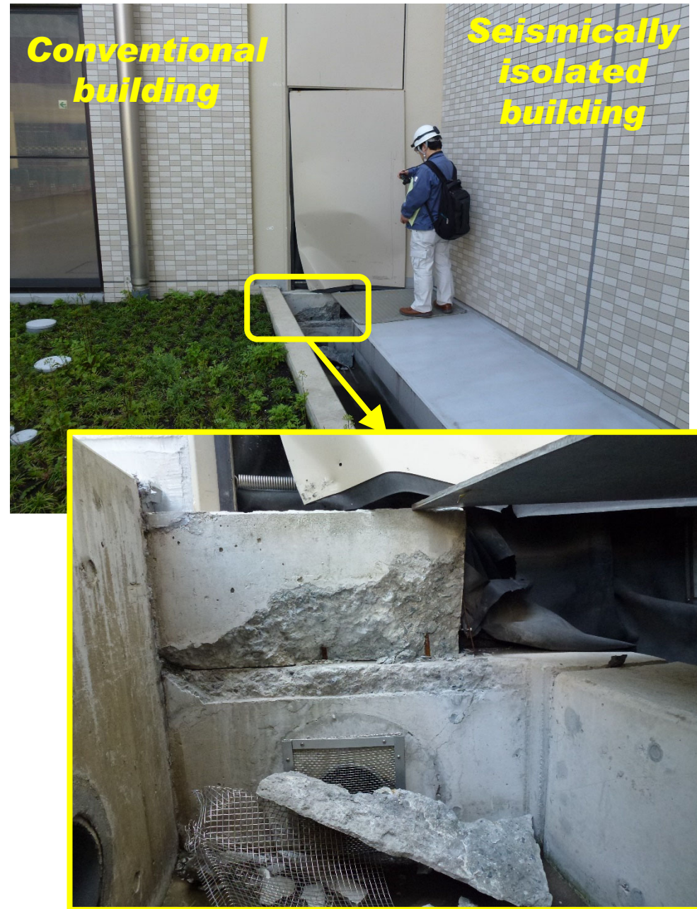
Damage of Expansion Joint
