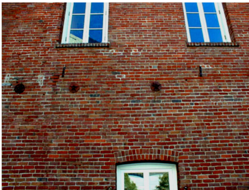
Figure E-54 Two existing anchors above three new wall anchors at floor line using decorative washer plates.
