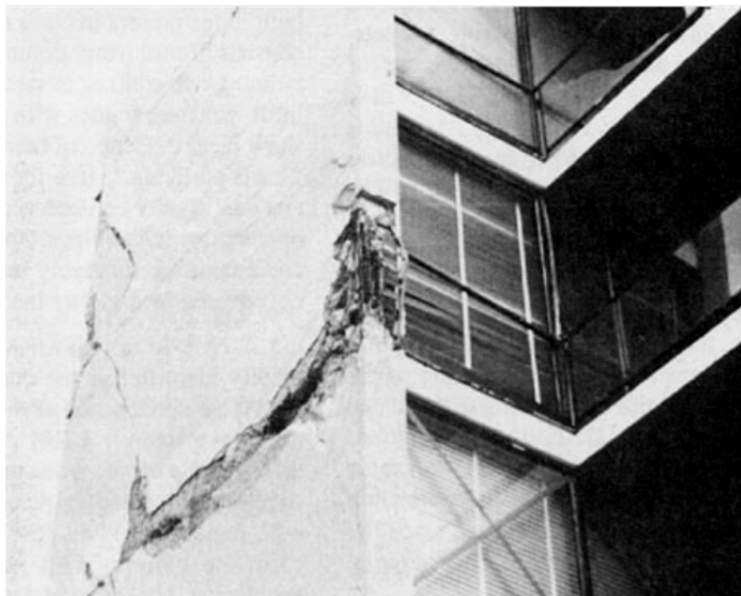
Figure E-21 Close-up of exterior shear wall damage during a major earthquake.
