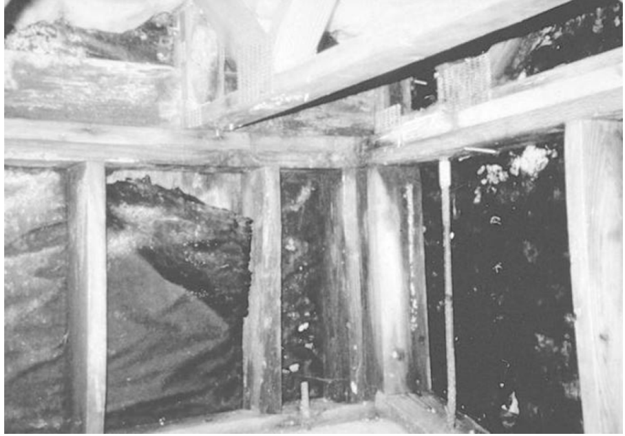
Figure F-1 Wood decay in cripple wall.
