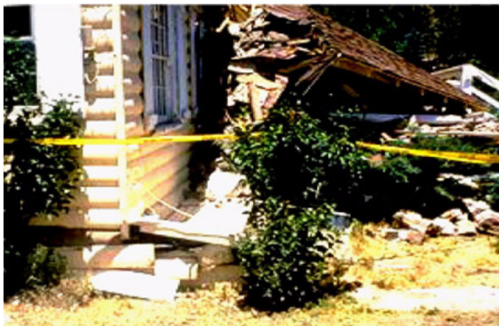
Figure G-6 Collapsed cripple stud walls dropped this house to the ground, 1992 Landers and Big Bear earthquakes.
