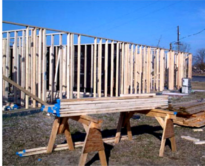
Figure E-5 Stud wall, wood framed house.
