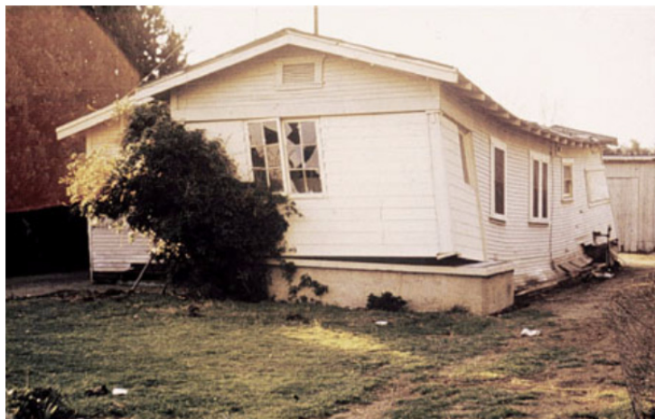
Figure G-5 House that slid off foundation, 1994 Northridge earthquake.
