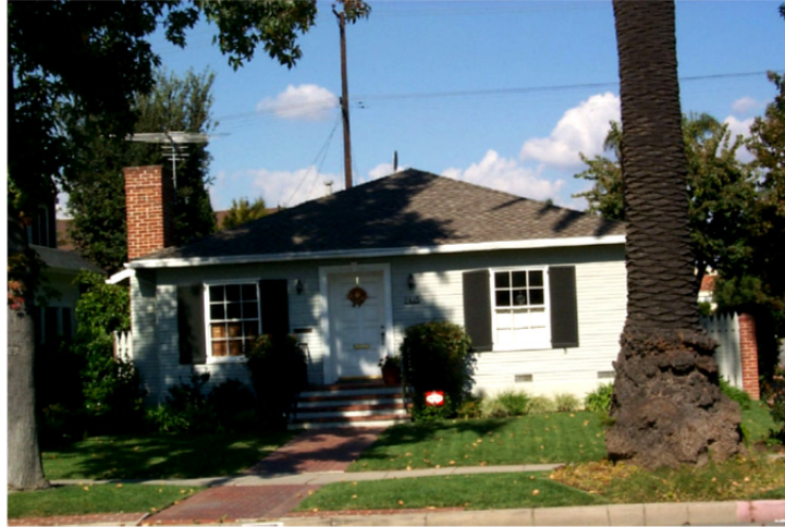
Figure E-1 Single family residence (an example of the W1 identifier, light wood frame single- or multiple-family dwellings of one or more stories in height).
