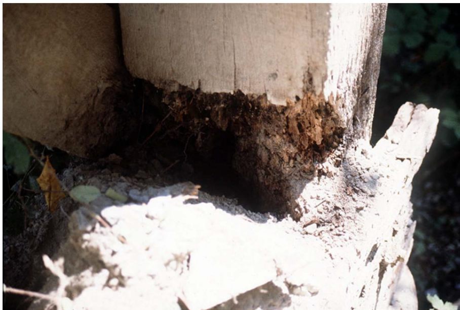
Figure F-3 Rotted timber column.
