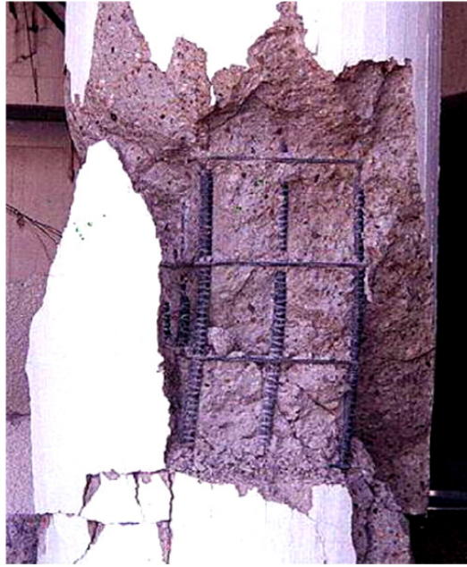
Figure E-26 Example of ductile reinforced concrete column, 1994 Northridge earthquake; horizontal ties would need to be closer for greater demands.
