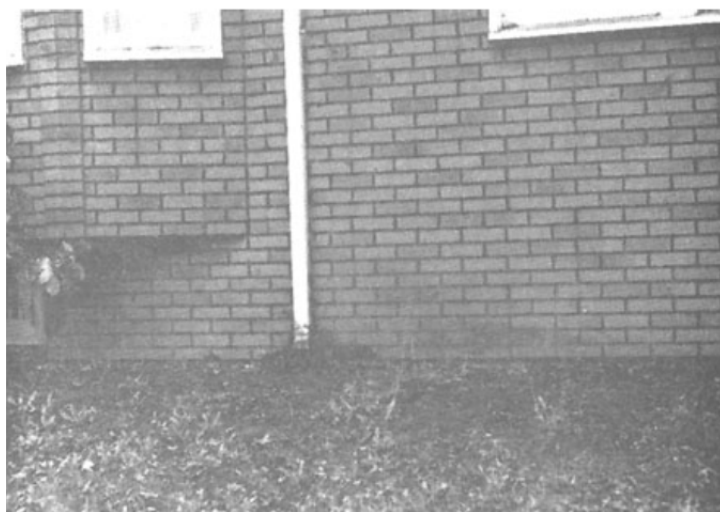
Figure D-16 Asphalt siding with brick pattern.
