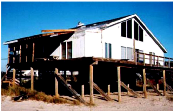
Figure E-7 Timber pole framed house.
