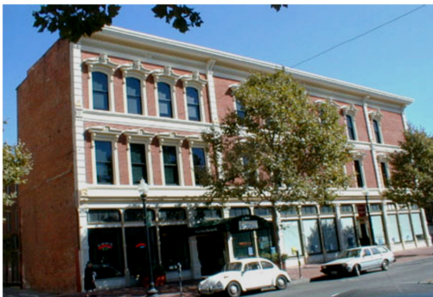
Figure E-50 West Coast URM bearing wall building.
