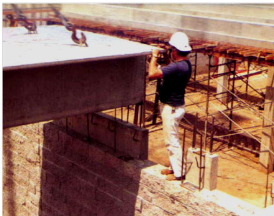
Figure E-43 Example of precast double “T” section during installation.
