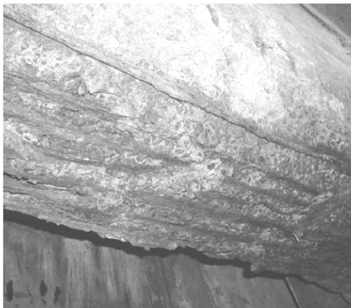
Figure F-6 Exposed reinforcing steel.
