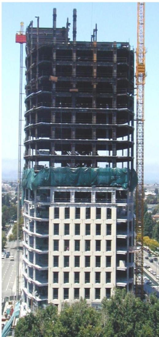
a. Building above is a high-rise steel dual system: moment frame (heavy columns and beams on upper façade) with bracing around elevator core. Fireproofing is being applied to steel at mid-height (inside the shroud) and precast façade elements are being attached to frame in lower stories.
