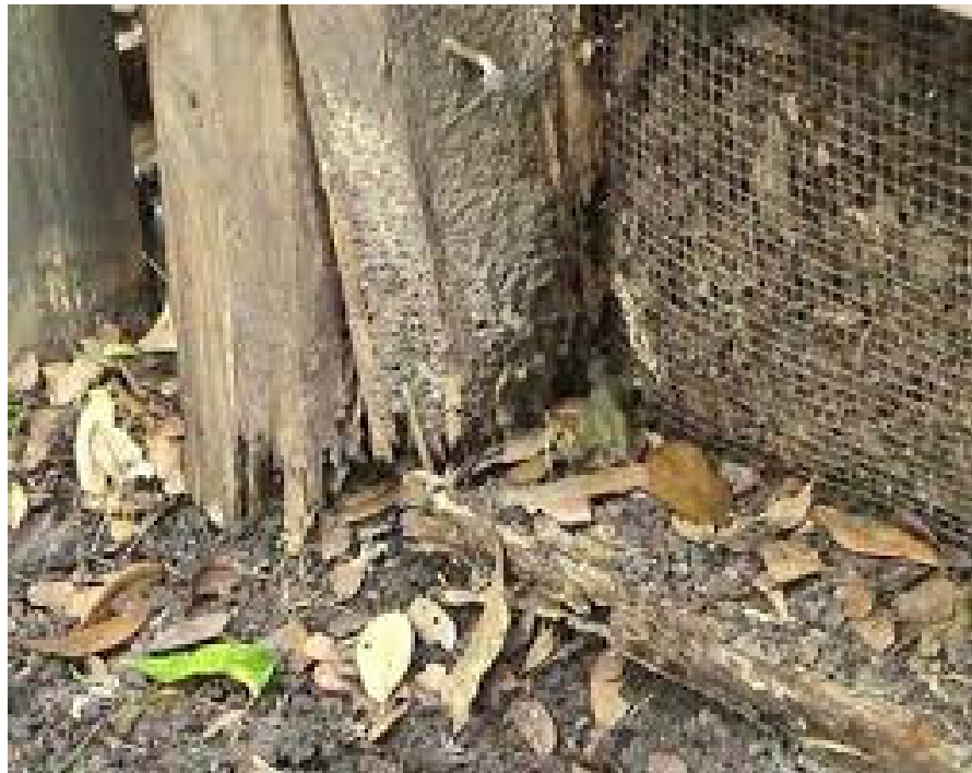
Figure F-2 Damaged wood post.
