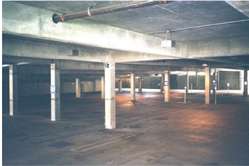
Figure 3-43 Interior view showing concrete columns and girders with no identifiable shear walls, which indicates a concrete moment frame (C1).
