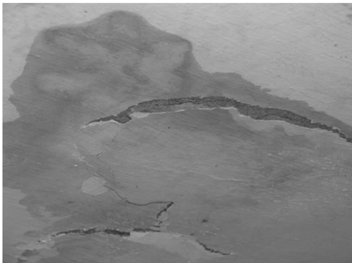
Figure F-5 Spalled concrete cover.
