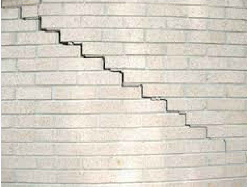
Figure F-8 "Stair-step" cracking.
