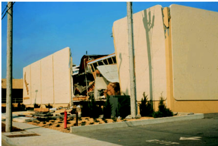
Figure E-38 Result of failure of the roof beam anchorage to the wall in tilt-up building.
