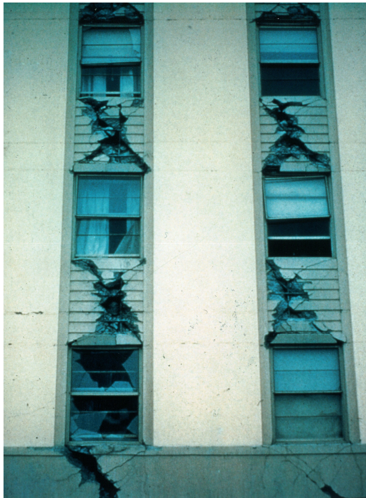
Figure E-30 Tall concrete shear wall building; walls connected by damaged spandrel beams.
