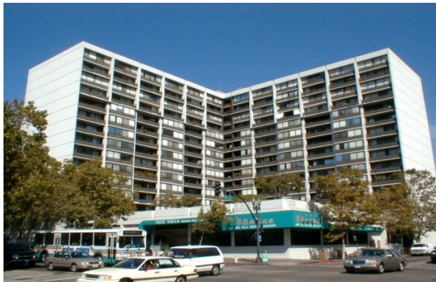
Figure 3-33 Building with a plan irregularity with two wings meeting at right angles.
