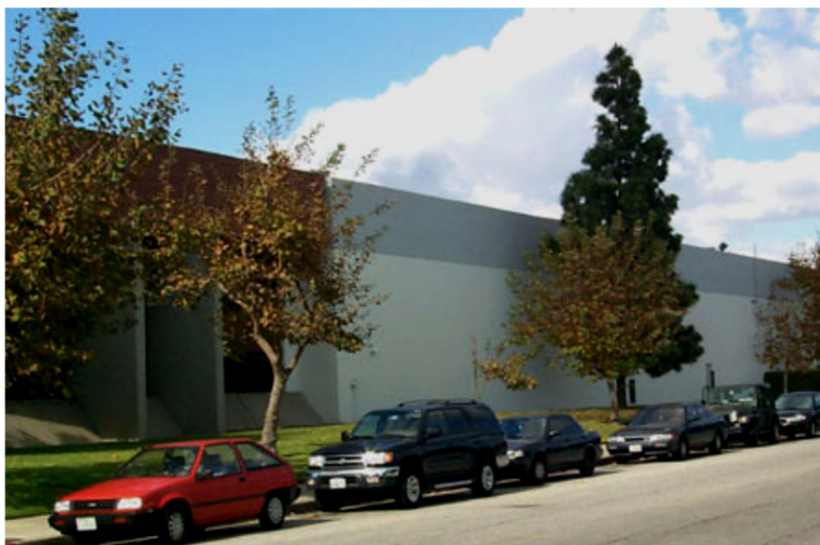
Figure E-35 Tilt-up industrial building, 1970s.
