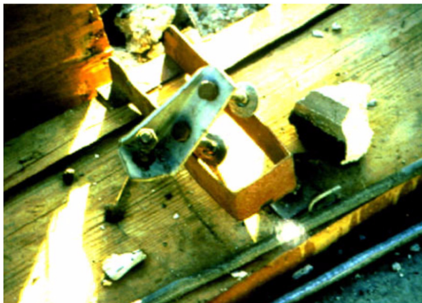
Figure E-37 Tilt-up construction anchorage failure.
