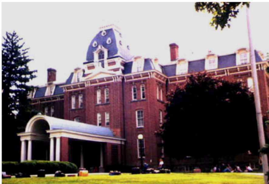
Figure E-49 East Coast URM bearing wall building.
