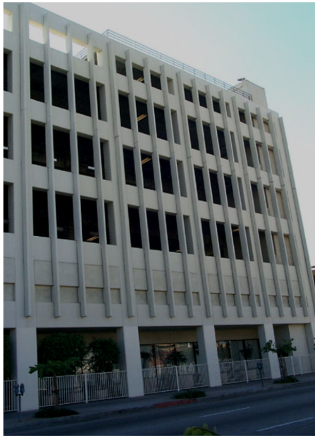
Figure E-27 Concrete moment-resisting frame building (C1) with exposed concrete, deep beams, wide columns (and with architectural window framing).
