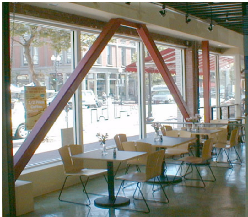
Figure E-16 Use of a braced frame to rehabilitate an unreinforced masonry building.
