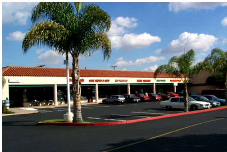
Figure E-3 Larger wood framed structure, typically with room-width spans (W2, commercial and industrial wood frame buildings greater than 5,000 square feet).
