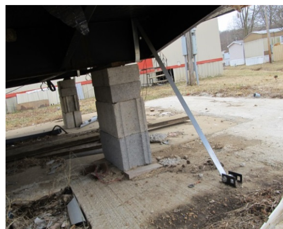
Figure 3-1 Examples of flood and wind tie-down systems for manufactured housing.
