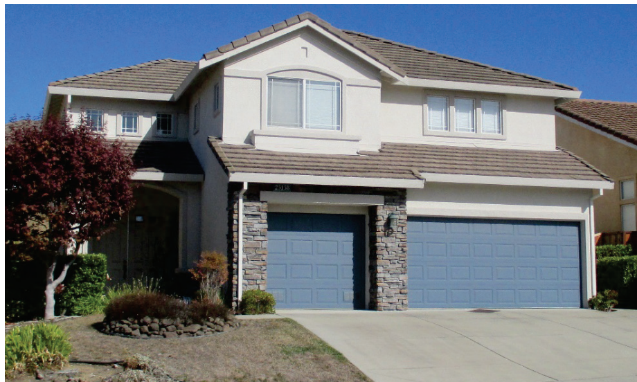
Figure 12-2 Typical L-shaped living-space-over-garage dwelling.
