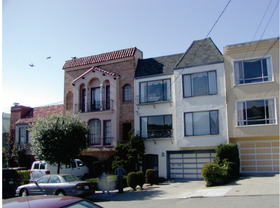
Figure 12-1 Typical rectangular living-space-over-garage dwelling.
