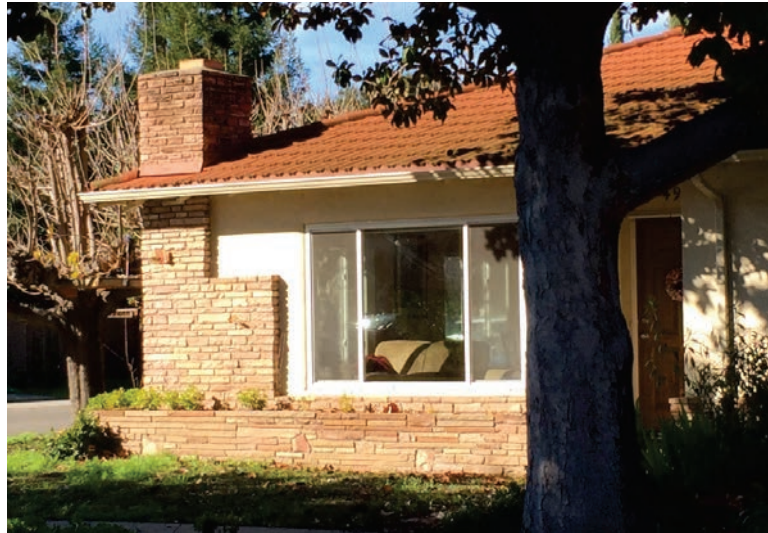
Figure 10-1 Example of ineligible chimney—corner construction with plan dimension greater than 40 inches. (Photo by authors).
