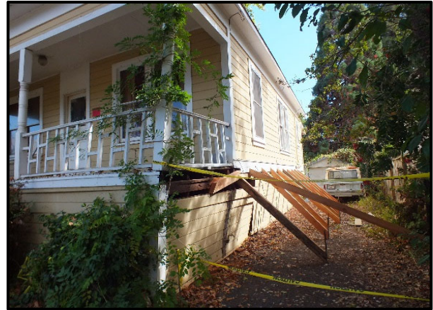
Figure 1: House with cripple walls damaged in the South Napa earthquake. Temporary bracing has been installed to provide stability and prevent collapse. Photo credit: Estructure.
