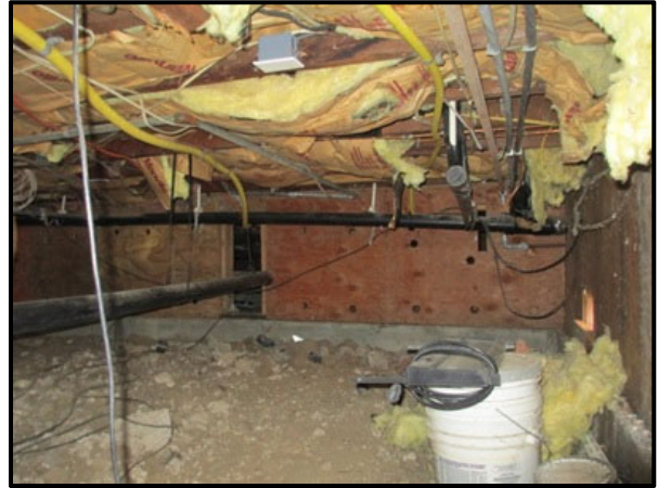
Figure 2: Cripple wall with plywood strengthening that was undamaged in the South Napa earthquake. Photo credit: ZFA Structural Engineers.
