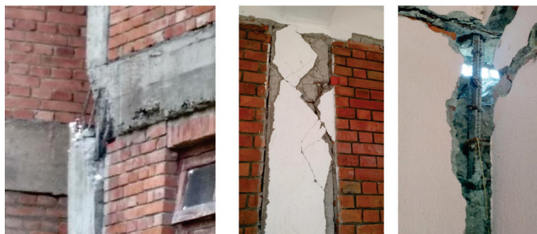
Figure O-23 Damage to an infilled frame building, showing severely damaged columns, but no collapse. Infill panels are likely carrying significant portion of the gravity loads (Bose et al., 2017).
