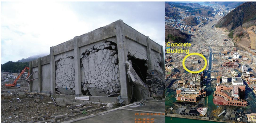
Figure 5. Concrete wall failure due to internal pressurization (left) and building location (right)
