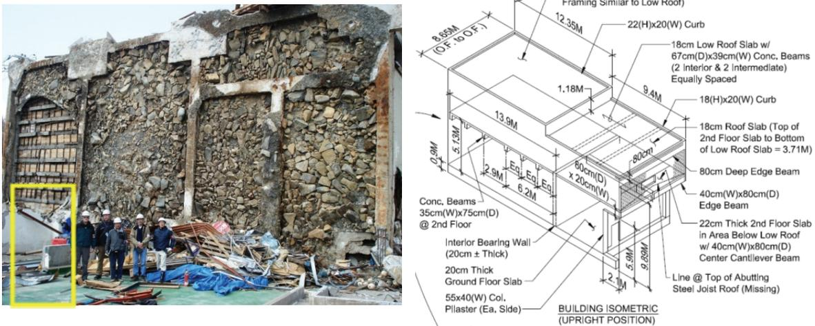
Figure 2. Onagawa uplifted and overturned 2-story RC building – floated over low wall in box
