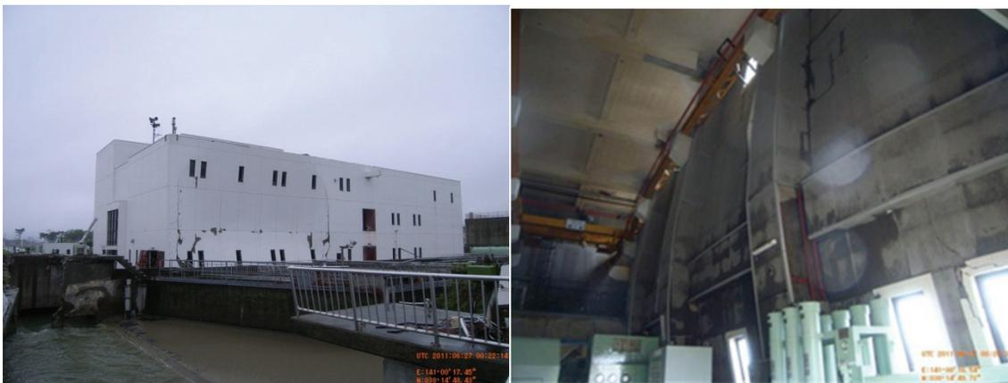
*Figure 9. Ocean-facing reinforced concrete wall at the Minami Gamou Wastewater Treatment Plant pump station building damaged by direct strike from tsunami bore (a) exterior view, (b) interior view*
