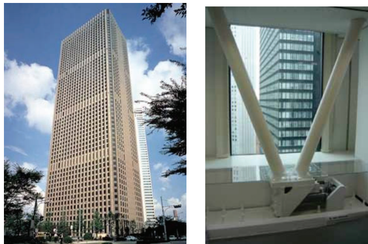
Figure 5. (Left) Picture of Shinjuku Center Building, and (right) dampers installed in 2009 (from EERI Newsletter, 2012).
