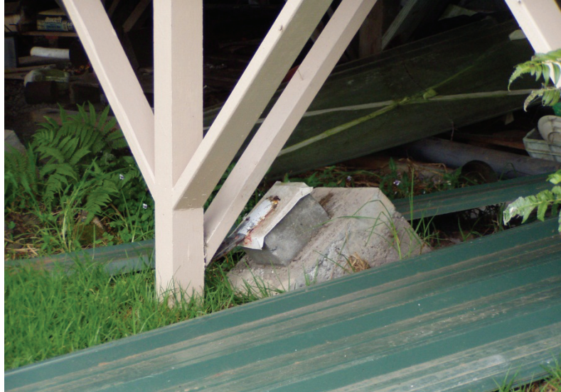
Figure 3. Seismic performance at discontinuous footings. This foundation type would result in 4.2 penalty points being assigned, reducing the Structural Score
