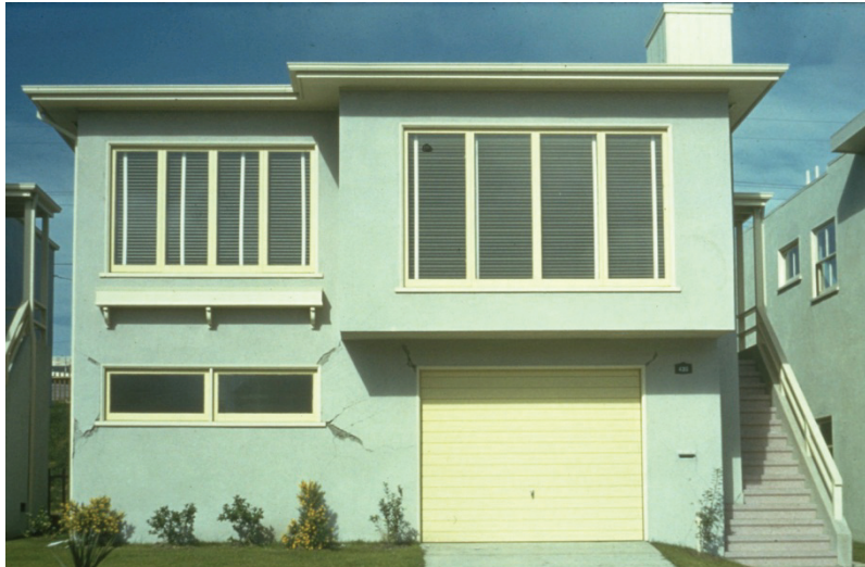
Figure 5. Dwellings are vulnerable where little bracing wall is provided at garage doors
