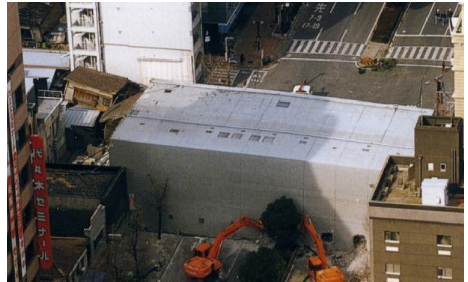
Photo. 2 Over turned building
