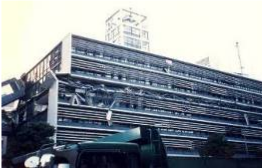
Kobe city hall after 1995 Kobe EQ
