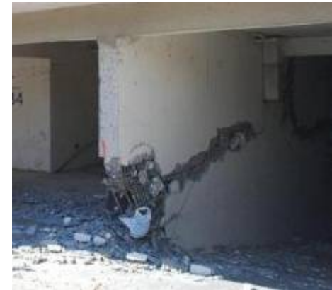
Shearwall damage in 2010 Chili EQ (EERI, 2010)
