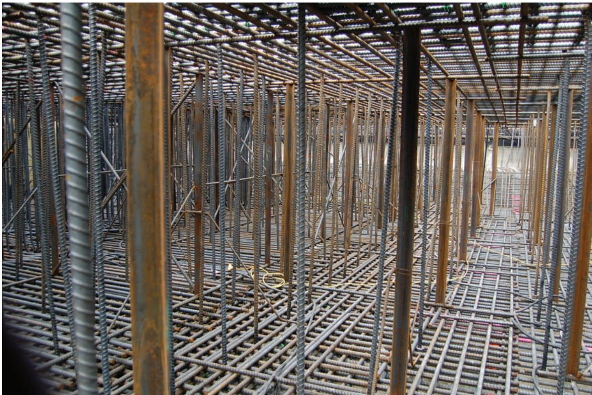
Figure 11-1 – Vertical reinforcement and steel angle standees.
