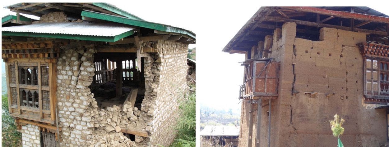
Figure 2. Vernacular stone masonry (left) and rammed earth (right) buildings showing types of damage many such buildings suffered in the 2009 and 2011 earthquakes, respectively. (Photo credits Department of Disaster Management, GeoHazards International)
