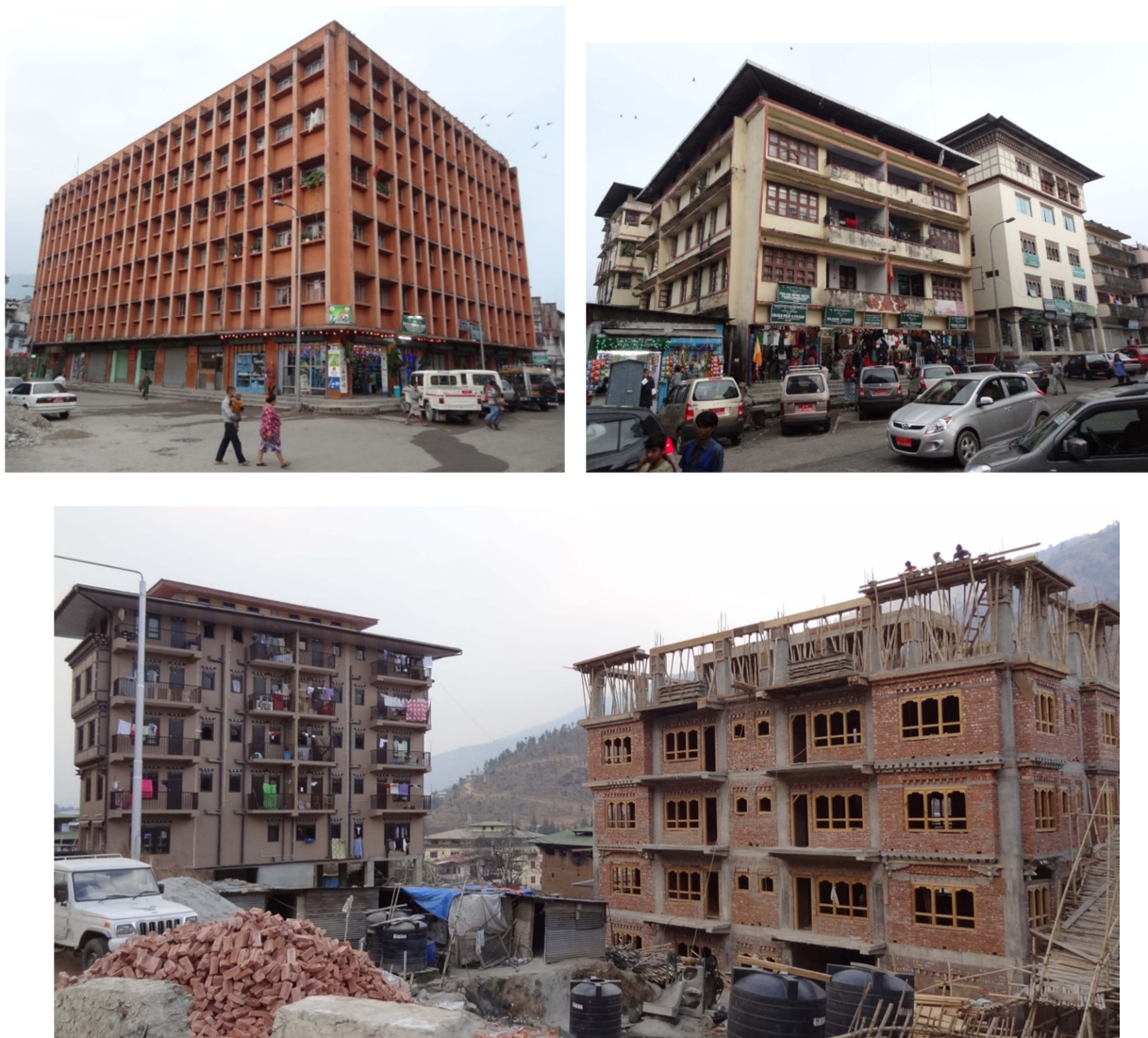
Figure 3. Older reinforced concrete buildings in Phuentsholing (top); new reinforced concrete frame buildings in Thimphu (bottom); (Photo credits Janise Rodgers, GeoHazards International).
