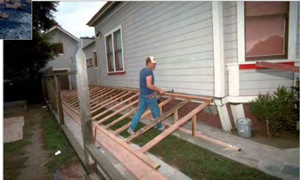
Photo by Bay Area Retrofit
