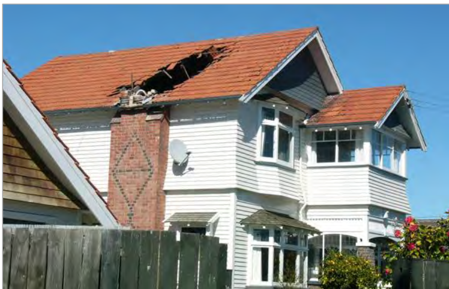
Photo from Element Roofing, 2010 Canterbury Earthquake, M7.1
