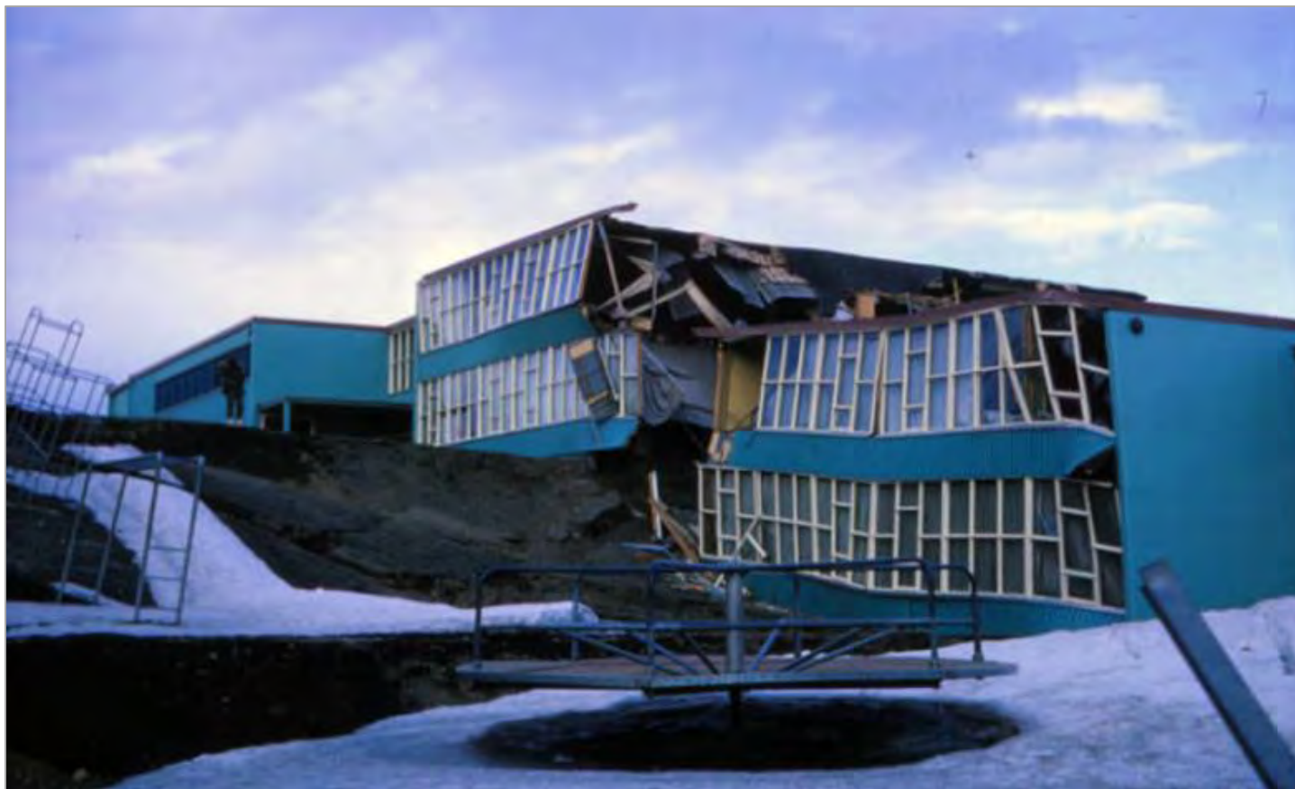
Government Hill Elementary, Anchorage, Alaska - 1964 Courtesy of Univ. of Alaska Anchorage, Special Collections
