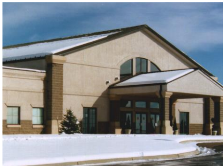
Metal building system with fallen snow on the roof.
