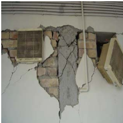
Photo 21: Shear crack in column
