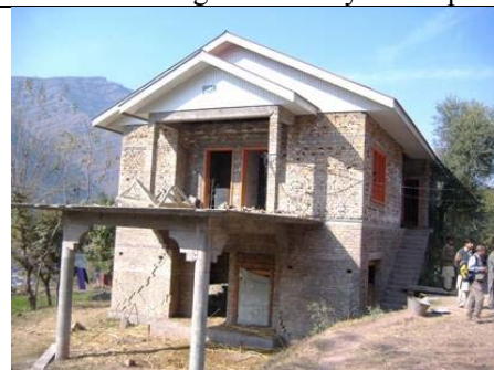
Photo 4: Severe Damage to Primary Structural System
