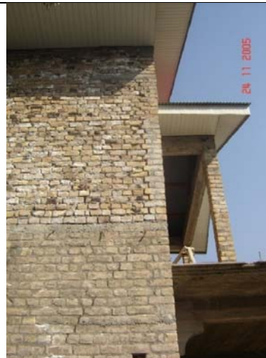
Photo 6: Moderate corner separation
