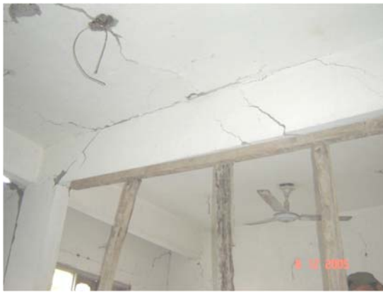
Photo 19: Shear cracks in beam near to support and at mid span
