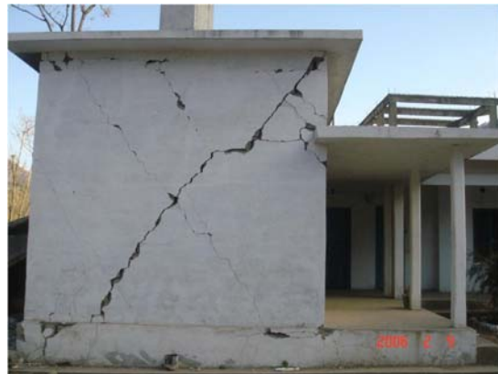
Photo 8: Diagonal cracking of solid wall
