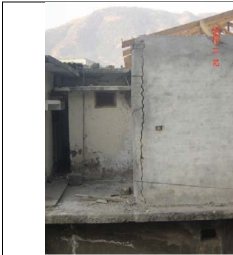
Photo 5: Heavy corner separation
