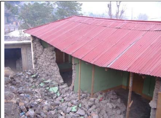
Photo 10: Out of plane failure of stone wall
