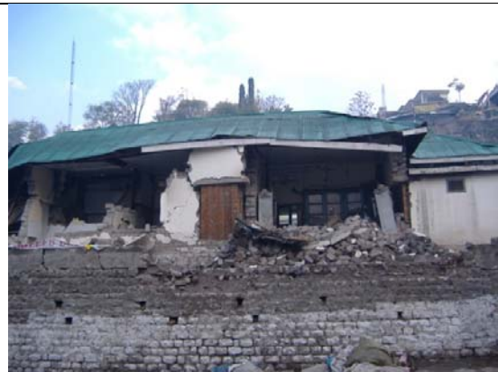
Photo 11: Out of plane failure of block wall
