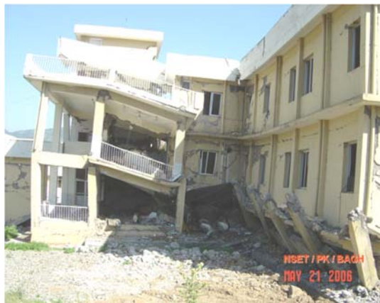
Photo 18: Earthquake damage due to soft story
