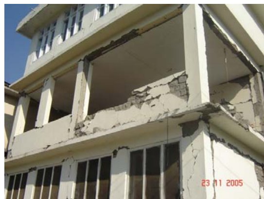
Photo 24: Extreme Damage to Infill wall
