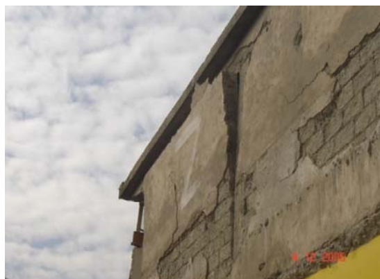
Photo 23: Moderate-Heavy Damage to Infill wall
