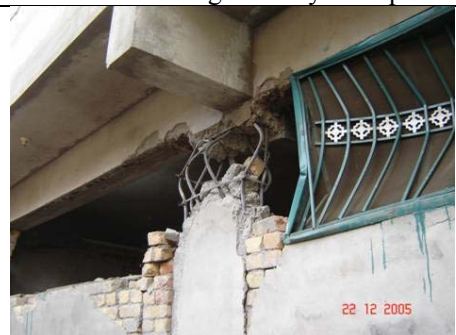
Photo 3: Severe Damage to Primary Structural System
