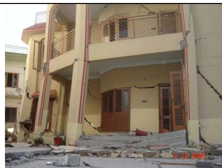
Photo 2: Building with a story out of plumb
