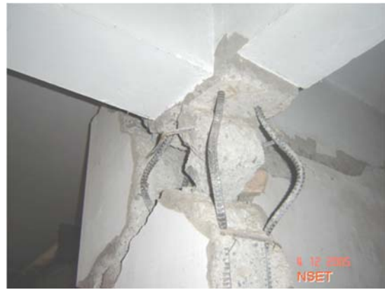
Photo 22: Buckling of column bars
