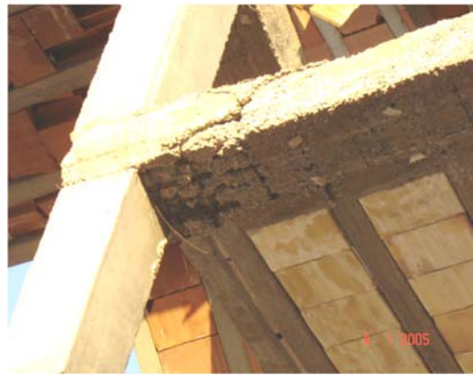
Photo 20: Shear crack in beam near to support
