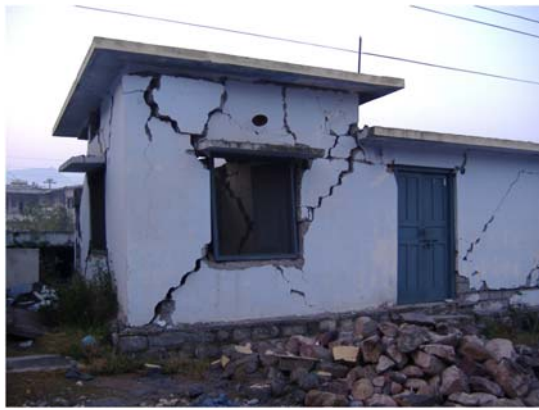
Photo 7: Diagonal cracking of masonry piers starting from corner of openings
