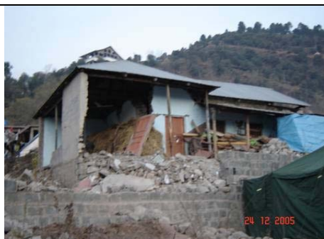
Photo 1: Building Partially Collapsed
